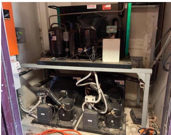
Line ID 46: External, Office Building, Ground Floor, Plant Room, Compressors, R404A Refrigerant - Non ODS Refrigerant
