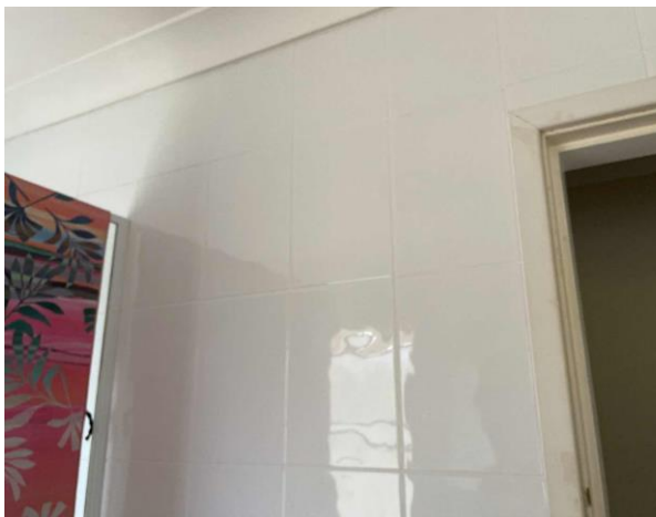
Line ID 29: Internal, Private Residence, Ground Floor, Bathroom, Behind Ceramic Tiles, Fibre Cement Sheeting - Suspected Asbestos
