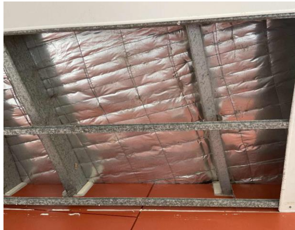
Line ID 43: Internal, Recreation Hall, Ground Floor, Underside of Roof, Sarking Insulation - Suspected SMF
