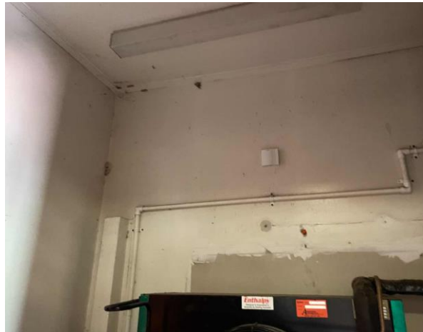
Line ID 26: Internal, Office Building, Ground Floor, Plant Room, Wall Lining, Fibre Cement Sheeting - Chrysotile Asbestos Detected
