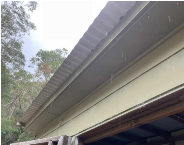
Line ID 1: External, Chemicals Storage Shed, Ground Floor, Eaves to Entrance Side of Shed, Compressed Cement Sheetting - No Asbestos Detected
