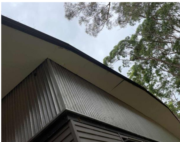
Line ID 11: External, Recreation Hall, Ground Floor, Eaves, Fibre Cement Sheetting - Suspected Asbestos
