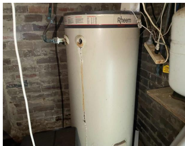
Line ID 35.1: External, Private Residence, Ground Level, North Elevation of Building, Hot Water Heater, Internal Insulation - Suspected SMF
