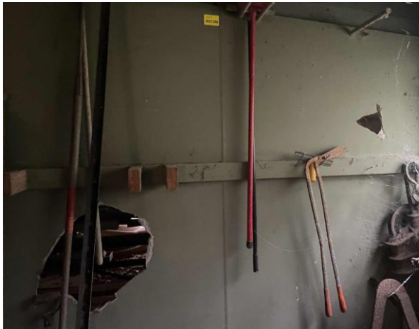
Line ID 19: Internal, Maintenance Shed, Ground Floor, Dividing Wall, Fibre Cement Sheet - No Asbestos Detected
