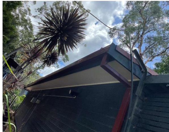
Line ID 16: External, Visiting Teachers Residence, Ground Floor, Eaves, Fibre Cement Sheetting - Suspected Asbestos
