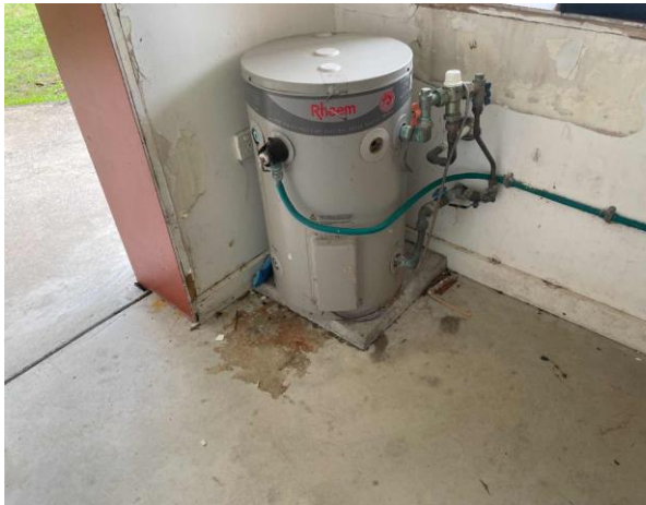
Line ID 42: Internal, Recreation Hall, Ground Floor, Tap Room, Hot Water Heater, Internal Insulation - Suspected SMF
