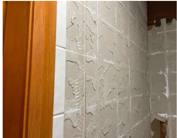
Line ID 20: Internal, Manager on Call House, Ground Floor, Ensuite Bathroom, Behind Ceramic Tiles, Compressed Cement Sheetting - No Asbestos Detected
