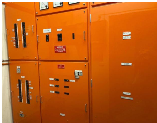
Line ID 6: External, Office Building, Ground Floor, Within Office, Main Switchboard and Redundant Fuses, HRC Fuses - Suspected Asbestos
