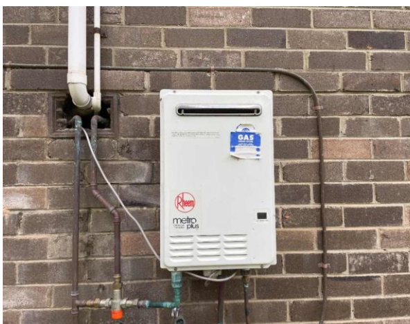
Line ID 35: External, Private Residence, Ground Level, North Elevation of Building, Hot Water Heater, Internal Insulation - Suspected SMF
