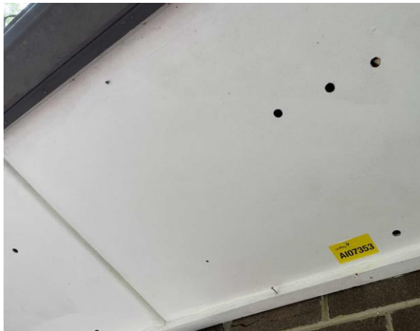
Line ID 7: External, Private Residence, Ground Level, Eaves, Fibre Cement Sheetting - Chrysotile and Amosite Asbestos Detected
