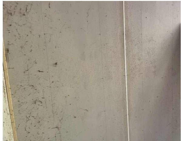
Line ID 22: Internal, Manager on Call House, Ground Floor, South-East Subfloor, Wall Lining, Fibre Cement Sheetting - No Asbestos Detected
