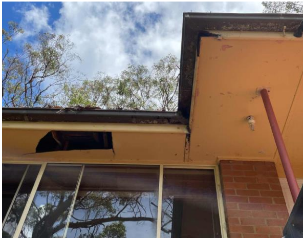
Line ID 15: External, Stone Lodge, Ground Floor, Eaves to Western Building, Fibre Cement Sheetting - Suspected Asbestos
