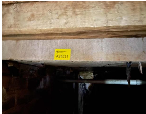
Line ID 10: External, Private Residence, Ground Level, Within Subfloor, Packing Material Under Stairwell, Fibre Cement Sheet - Chrysotile Asbestos Detected
