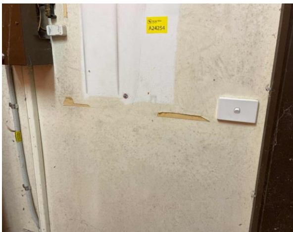
Line ID 5: External, Office Building, Ground Floor, Switchboard Room, Wall Lining, Fibre Cement Sheetting - Chrysotile Asbestos Detected
