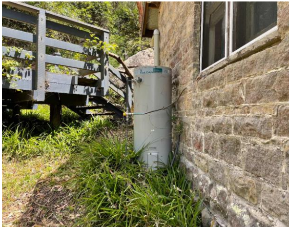
Line ID 36: External, Stone Lodge, Ground Floor, Eastern Building, Hot Water Unit, Internal Insulation - Suspected SMF
