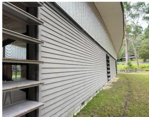
Line ID 12: External, Recreation Hall, Ground Floor, Walls, Weatherboard Cladding, Compressed Cement Sheetting - No Asbestos Detected
