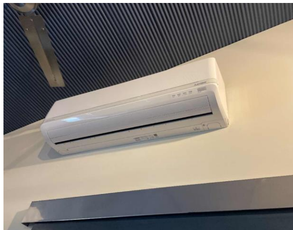
Line ID 45: External, Holiday Units 1-4, Ground Floor, Throughout, Wall Mounted Air Conditioning Unit, R410A Hydrofluorocarbon (HFC) - Non ODS Refrigerant
