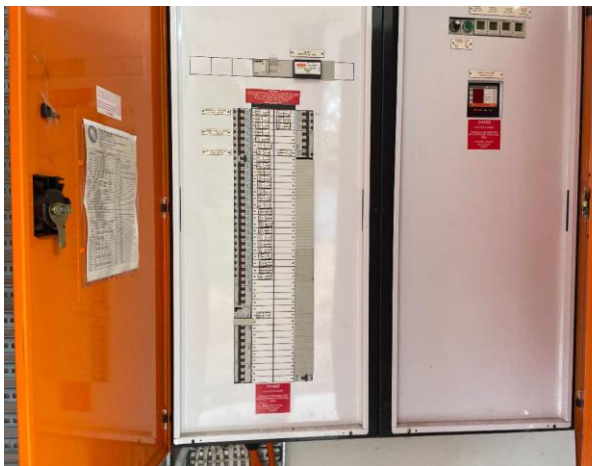
Line ID 33: Internal, Recreation Hall, Ground Floor, Main Switchboard Cupboard, HRC Fuses - Suspected Asbestos
