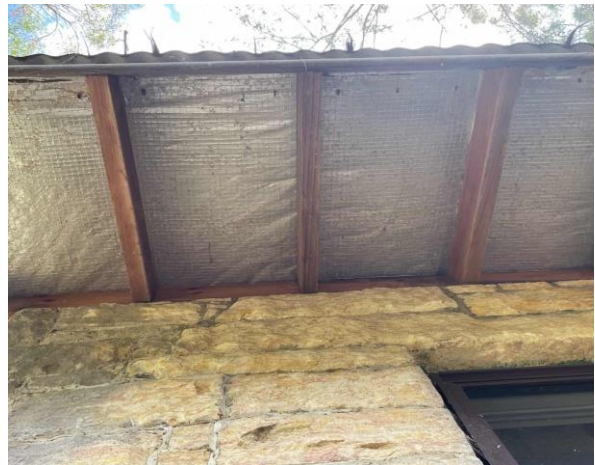
Line ID 37: External, Stone Lodge, Ground Floor, Eastern Building, Underside of Roof, Sarking Insulation - Suspected SMF
