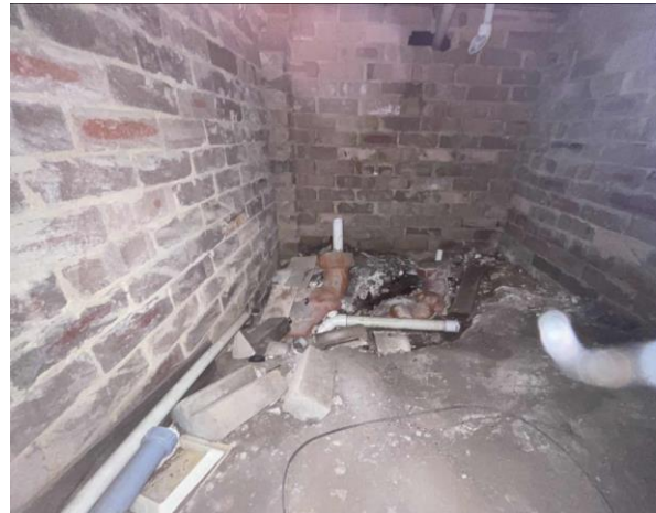
Line ID 8: External, Private Residence, Ground Level, Subfloor, Debris Throughout, Fibre Cement Sheet - Chrysotile Asbestos Detected
