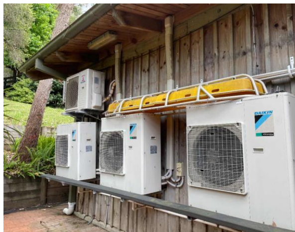
Line ID 47: External, Office Building, Ground Floor, South of Building, Air Conditioning Unit, R410A Hydrofluorocarbon (HFC) - Non ODS Refrigerant
