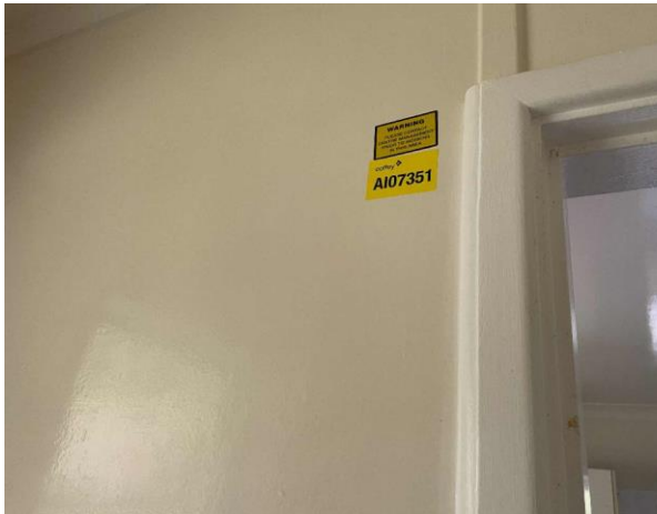
Line ID 31: Internal, Private Residence, Ground Floor, Laundry, Wall Lining, Fibre Cement Sheetting - Chrysotile Asbestos Detected
