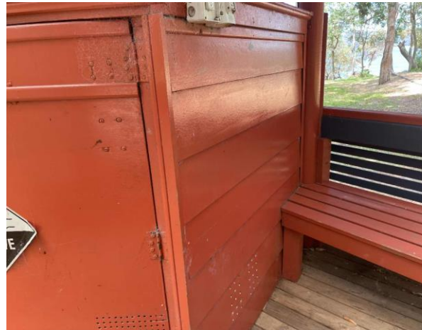
Line ID 14: External, Rotunda Canopy, Ground Floor, Walls Within Canopy Area, Compressed Cement Sheetting - No Asbestos Detected
