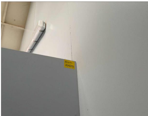
Line ID 27: Internal, Pool Area, Ground Floor, Female and Male Bathrooms, Wall Lining and Cubicle Partitions, Compressed Cement Sheeting - No Asbestos Detected
