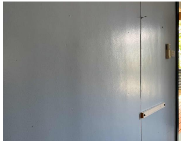
Line ID 24: Internal, Meeting Room, Ground Floor, Aboriginal Museum, Wall Lining, Fibre Cement Sheetting - No Asbestos Detected
