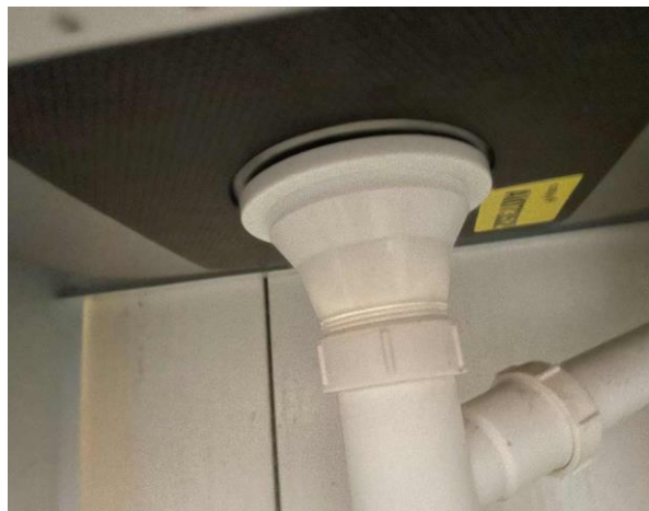
Line ID 30: Internal, Private Residence, Ground Floor, Laundry Room, Under Sink, Sink Pad, Bituminous Membrane - No Asbestos Detected
