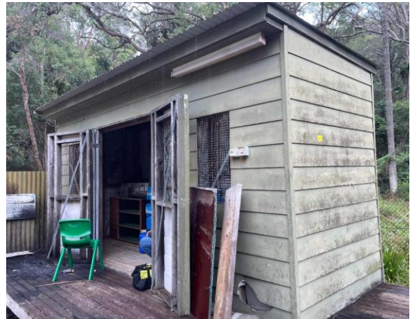
Line ID 2: External, Chemicals Storage Shed, Ground Floor, Walls, Weatherboard Cladding, Compressed Cement Sheetting - No Asbestos Detected
