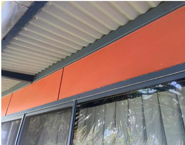
Line ID 3: External, Holiday Units 1-4, Ground Floor, Fascia Panels, Fibre Cement Sheetting - No Asbestos Detected
