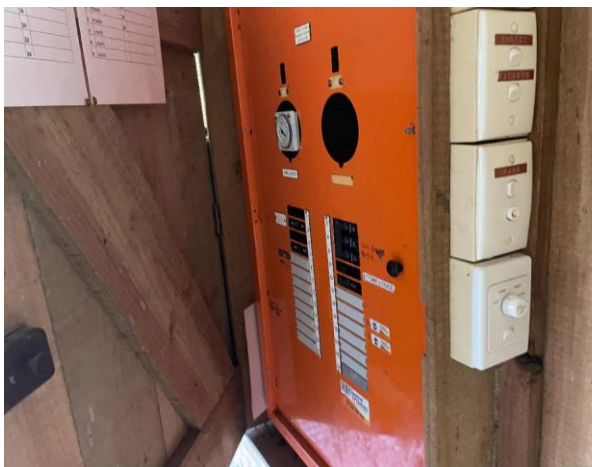
Line ID 17: Internal, Accommodation Lodges, Ground Floor, Within Wall Mounted Switchboard Cupboards, HRC Fuses - Suspected Asbestos
