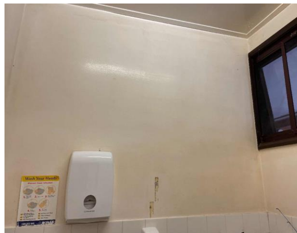
Line ID 18: Internal, Dining Hall, Ground Floor, Laundry Room, Wall Lining, Fibre Cement Sheetting - Chrysotile Asbestos Detected
