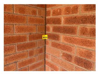
Line ID 14: External, Girrawaa Lodge, Elevations, Brickwork, Vertical Joints Throughout, Construction Joint Mastic - No Asbestos Detected
