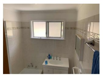
Line ID 76: Internal, General Managers Residence, Bathroom/Shower, Wall Lining, Compressed Cement Sheet -Chrysotile Asbestos Detected
