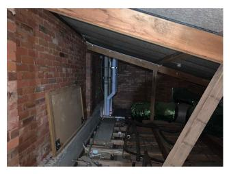
Line ID 70: Internal, Dining Hall Complex, Level 1, West Ceiling Space, South Portion of Ceiling Space, Moulded Fibre Cement - Chrysotile Asbestos Detected
