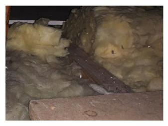
Line ID 157: Internal, General Managers Residence, Ceiling Space Throughout, Ceiling Space, Representative Image of Loose Insulation Batts - Suspected SMF
