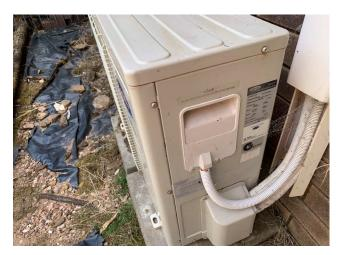
Line ID 198: External, General Managers Residence, East Side, Garden Area, Refrigerant Gas to AC Split System, R410A Hydrofluorocarbon (HFC) - Non ODS Refrigerant
