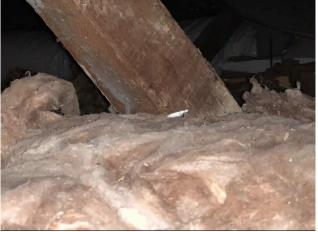
Line ID 149: Internal, Client Services Coordinator Residence, Ceiling Space Throughout, Ceiling Lining, Loose Insulation Batts - Suspected SMF
