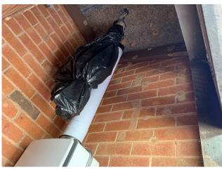
Line ID 115: Internal, Meroo and Yarraman Lodge, Utilities Closets, SW Closet, Domestic Hot Water System, Moulded Cement Flue - Chrysotile Asbestos Detected
