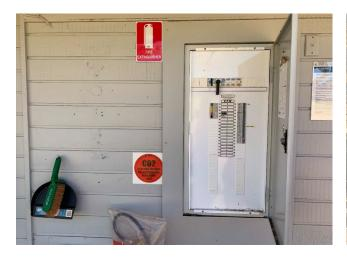
Line ID 34: External, Meroo and Yarraman Lodge, DB3 Cabinet Located SW of Building, Bituminous Electrical Backing Board - Suspected Asbestos
