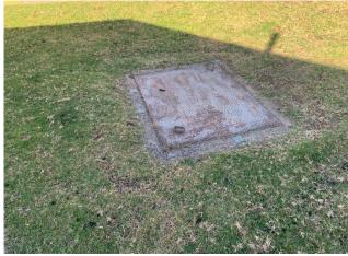
Line ID 26: External, Loading Dock Building, Elevations, West Side, Cement Communication Pit Lining, Fibre Cement Sheet - Chrysotile & Amosite Asbestos Detected
