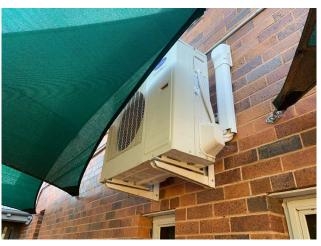
Line ID 197: External, Dining Hall Complex, North Side of Complex, Wall Mounted, Refrigerant Gas to 'Carrier' AC Split System, R22 Hydrochlorofluorocarbon (HCFC) - ODS Refrigerant
