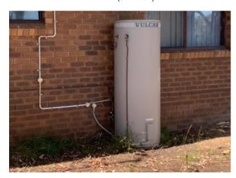
Line ID 139: External, Client Services Coordinator Residence, Residence, West Side, Rheem Domestic Hot Water System, Internal Insulation Material - Suspected SMF
