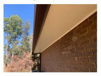
Line ID 39: External, Services Coordinator Residence, Perimeter of Residence, Eaves Lining, Compressed Cement Sheet - Chrysotile Asbestos Detected
