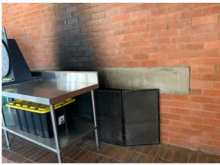
Line ID 63: Internal, Dining Hall Complex, Ground Level Dining Room And Middle Corridor, Within Fire Place and Chimney, Flue, Moulded Fibre Cement - Suspected Asbestos
