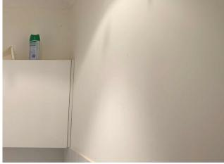
Line ID 79: Internal, General Managers Residence, Toilet, Wall Lining, Compressed Cement Sheet - Chrysotile Asbestos Detected
