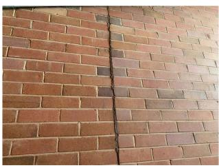
Line ID 61.1: Internal, Dining Hall Complex, Elevations, Vertical Wall Joints Throughout, Construction Joint Mastic - Chrysotile Asbestos Detected
