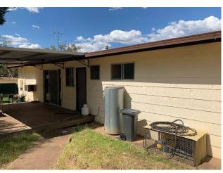
Line ID 7: External, Client Services Coordinator Residence, Residence, Eaves, Compressed Cement Sheet - Chrysotile Asbestos Detected
