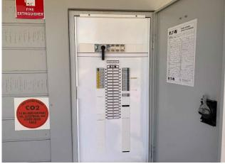
Line ID 15: External, Goonal and Mullion Lodge, Elevations, DB4 Cabinet Located SW Corner of Building, Bituminous Backing Board - Suspected Asbestos
