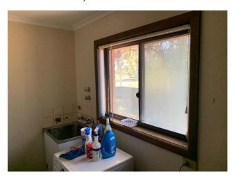
Line ID 122: Internal, Service Coordinator Residence, Laundry, NE Corner of Residence, Wall Lining, Compressed Cement Sheet - Chrysotile Asbestos Detected
