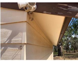
Line ID 5: External, Client Services Coordinator Residence, Garage, East and West Elevations, Eaves Lining, Compressed Cement Sheet - Chrysotile Asbestos Detected
