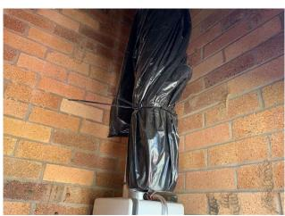
Line ID 105.1: Internal, Merinda and Curra Gurra Lodge, NE and SW Closets, Hot Water System, Formed Asbestos Cement Flue Pipe - Chrysotile & Amosite Asbestos Detected
