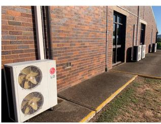
Line ID 193: External, Conference Room Building, North Side, Refrigerant Gas to LG AC Split System, R22 Hydrochlorofluorocarbon (HCFC) - ODS Refrigerant
