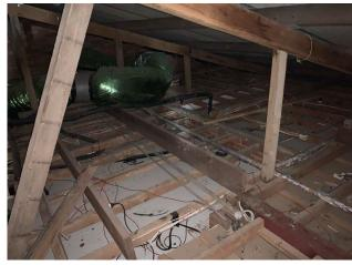
Line ID 154: Internal, Dining Hall Complex, Level 1, West Ceiling Space, South Ceiling Space, Flexible Ductwork Insulation - Suspected SMF
