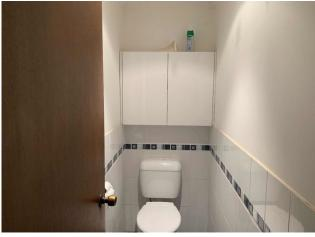
Line ID 123: Internal, Service Coordinator Residence, Toilet, Wall Lining, Compressed Cement Sheet - Chrysotile Asbestos Detected
