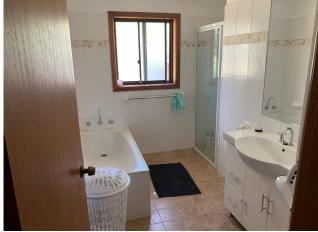
Line ID 119: Internal, Service Coordinator Residence, Bathroom/Shower, Wall Lining, Compressed Cement Sheet -Chrysotile Asbestos Detected
