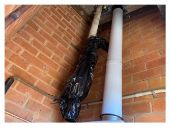
Line ID 106: Internal, Merinda and Curra Gurra Lodge, Utilities Closets, NE and SW Closets, in the Base Collar of Hot Water System Flues, Woven Rope - Chrysotile Asbestos Detected
