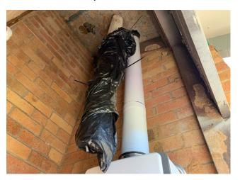
Line ID 81: Internal, Goonal and Mullion Lodge, Utilities Closets, NE And SW Closets, In Base Collar of Hot Water System Flues, Woven Rope - Chrysotile Asbestos Detected
