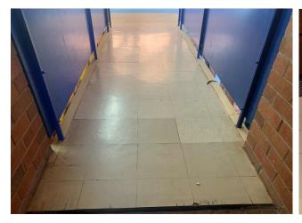
Line ID 67.1: Internal, Dining Hall Complex, Level 1 Throughout, Floor Covering, Vinyl Floor Tiles (Beige With Brown Fleck) - Chrysotile Asbestos Detected
