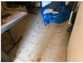
Line ID 101: Internal, Maintenance Workshop, Garage, Store Room, Cream Vinyl Floor Tiles - Chrysotile Asbestos Detected
