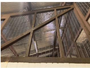
Line ID 161: Internal, Loading Dock Building, Internal, Ceiling Space, Ceiling Throughout, Sarking Insulation - Suspected SMF
