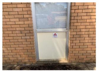
Line ID 28: External, Maintenance Workshop, Garage, Below South Window, Thick Infill Panel, Compressed Cement Sheet - Chrysotile Asbestos Detected
