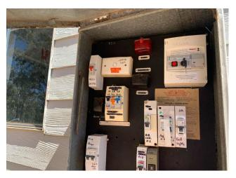
Line ID 21: External, Lakeside Cottages 1 & 2, South Side Cottage 1 in Electrical Box, Bituminous Electrical Backing Board - Chrysotile Asbestos Detected
