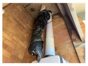
Line ID 105: Internal, Merinda and Curra Gurra Lodge, NE and SW Closets, Hot Water System, Formed Asbestos Cement Flue Pipe - Chrysotile & Amosite Asbestos Detected
