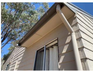
Line ID 22: External, Lakeside Cottages 1 & 2, Perimeter of Cottage 1, Eaves Lining - Sections above Windows, Compressed Cement Sheet - Chrysotile Asbestos Detected
