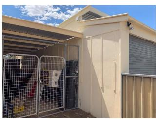
Line ID 136: External, Maintenance Workshop, Elevations, Garage Timber Barge Boards & West Wall of Workshop, Exterior Brown Paint - Lead Detected (0.1% w/w)
