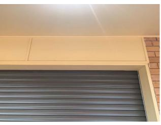
Line ID 138: External, Maintenance Workshop, Garage, Roller Door Frames, Eaves and Infill Panels and Timber Doors, Exterior White Paint - Lead Detected (0.2% w/w)
