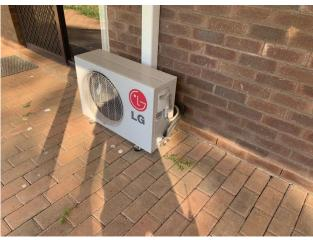
Line ID 210: External, Staff Lodge (Staff Residence), North Side of Building, Refrigerant Gas to AC System, R22 Hydrochlorofluorocarbon (HCFC) - ODS Refrigerant
