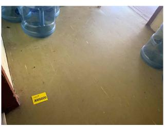
Line ID 97: Internal, Loading Dock Building, Hallway and Storage Room, Floor Covering, Green Vinyl Sheet - No Asbestos Detected
