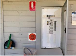
Line ID 31: External, Merinda and Curra Lodge, Elevations, DB3 Cabinet Located SW Corner of Building, Bituminous Electrical Backing Board - Suspected Asbestos
