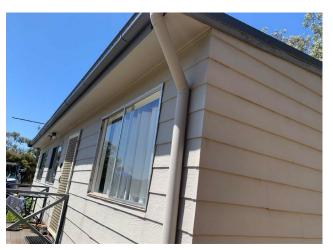
Line ID 24: External, Lakeside Cottages 1 & 2, Perimeter of Cottage 2, Eaves Lining - Sections above Windows, Compressed Cement Sheet - Chrysotile Asbestos Detected
