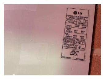
Line ID 190: External, Administration Complex, Elevations, North Side of Complex, Refrigerant Gas to The 'LG' AC Split System, R22 Hydrochlorofluorocarbon (HCFC) - ODS Refrigerant
