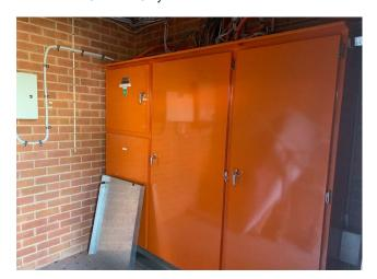
Line ID 72: Internal, Dining Hall Complex, Main Switch Room, Orange Metal Cabinets, Bituminous Electrical Backing Board - Suspected Asbestos
