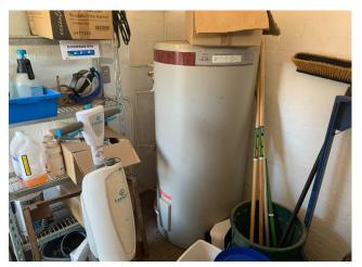
Line ID 155: Internal, Dining Hall Complex, Shower Room, Vulcan Hot Water System, Internal Insulation Material -Suspected SMF
