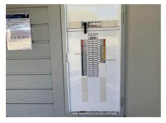
Line ID 46: External, Visiting Staff Rooms, Elevations, DB2 Cabinet Located SW Corner, Bituminous Backing Board -Suspected Asbestos
