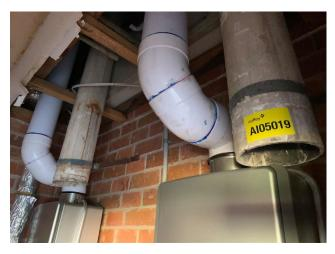
Line ID 74: Internal, Dining Hall Complex, West Hot Water Closet, Ceiling Area, Redundantly Pipes, Moulded Fibre Cement - Chrysotile Asbestos Detected
