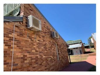
Line ID 207: External, Merinda and Curra Lodge, North and South Side and On Roof and Wall, Within 'LG' Split System, R22 Hydrochlorofluorocarbon (HCFC) - ODS Refrigerant
