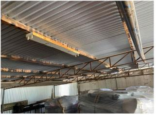
Line ID 170: External, Maintenance Workshop, Garage, East Eaves and Awnings, Twin Long Tube Light, Capacitor(s) - Suspected PCB
