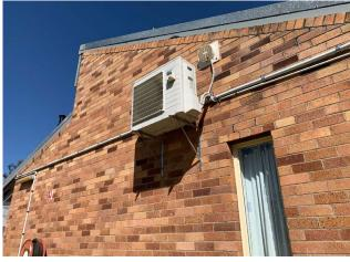
Line ID 206: External, Merinda and Curra Lodge, Elevations, North and South Elevations, Refrigerant Gas to The 'Daikin' AC Units, R22 Hydrochlorofluorocarbon (HCFC) - ODS Refrigerant
