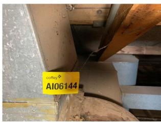
Line ID 69: Internal, Dining Hall Complex, Level 1, West Ceiling Space, Rigid Ductwork, Seems and Flanges, Mastic Sealant - No Asbestos Detected
