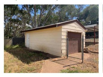
Line ID 6: External, Client Services Coordinator Residence, Garage, Wall Cladding, Compressed Cement Sheet -Chrysotile Asbestos Detected
