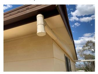
Line ID 8: External, Client Services Coordinator Residence, Residence, Wall Cladding, Compressed Cement Sheet -Chrysotile Asbestos Detected
