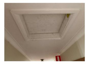
Line ID 55: Internal, Client Services Coordinator Residence, Hallway, Manhole Cover, Compressed Cement Sheet -Chrysotile & Amosite Asbestos Detected
