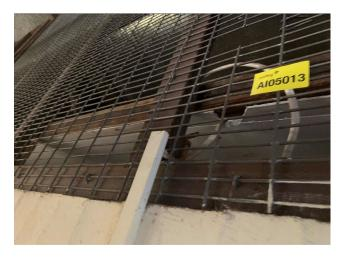
Line ID 98: Internal, Loading Dock Building, Ceiling Space, North Portion, Floor, Panelling, Compressed Cement Sheet -Chrysotile Asbestos Detected
