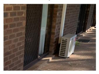
Line ID 211: External, Staff Lodge (Staff Residence), South Side of Building, Refrigerant Gas to 'LG' AC Split System, R22 Hydrochlorofluorocarbon (HCFC) - ODS Refrigerant
