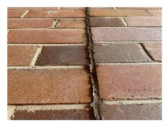
Line ID 61: Internal, Dining Hall Complex, Elevations, Vertical Wall Joints Throughout, Construction Joint Mastic - Chrysotile Asbestos Detected
