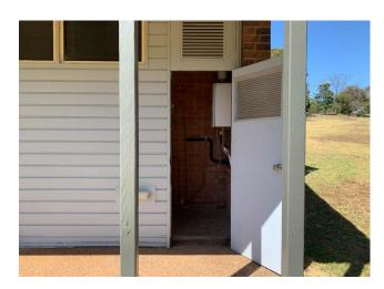
Line ID 169: Internal, Visiting Staff Rooms, Utilities Closets, NE and SW Closets, Rheem Hot Water System, Internal Insulation Material - Suspected SMF
