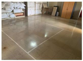
Line ID 50: Internal, Administration Complex, North Section Lower Level Supplies Area, Floor and Steps, Vinyl Floor Tiles Beige With Brown Fleck - Chrysotile Asbestos Detected
