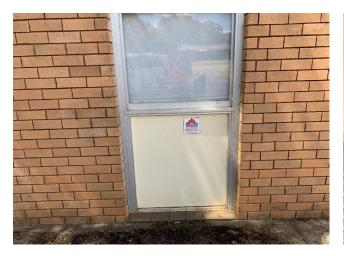
Line ID 137: External, Maintenance Workshop, Garage, Infill Panel Below South Window, Exterior Brown Paint - Lead Detected (0.1% w/w)
