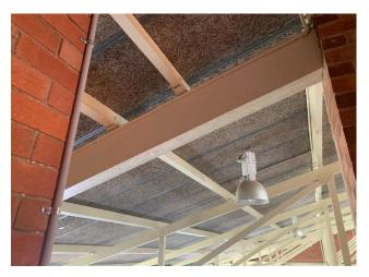
Line ID 151: Internal, Conference Room Building, Bulk Food Store and Bushcraft Centre, Ceiling Space Throughout, Underside of Roof Beneath Panels, Sarking Insulation -Suspected SMF
