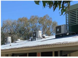
Line ID 212: External, Visiting Staff Rooms, Elevations, Located Adjacent Southern Enclosure, Refrigerant Gas to AC Unit, R22 Hydrochlorofluorocarbon (HCFC) - ODS Refrigerant
