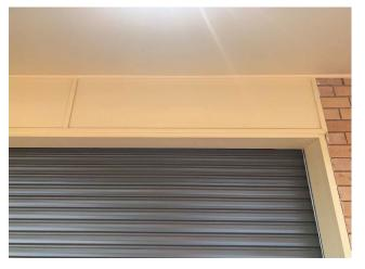
Line ID 30: External, Maintenance Workshop, Garage, Infill Panels above Roller Doors, Compressed Cement Sheet - Chrysotile Asbestos Detected
