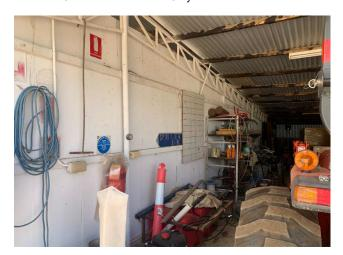
Line ID 102: Internal, Maintenance Workshop, Garage, Store Room, Wall Lining, Compressed Cement Sheet - Chrysotile Asbestos Detected
