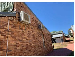
Line ID 208: External, Meroo and Yarraman Lodge, North and South Side and on Roof, Refrigerant Gas to AC System, R22 Hydrochlorofluorocarbon (HCFC) - ODS Refrigerant
