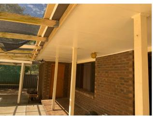
Line ID 38: External, Services Coordinator Residence, Elevations, East (Rear Entry) and West (Main Entry), Compressed Cement Sheet - Chrysotile Asbestos Detected
