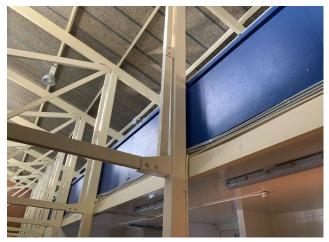
Line ID 66: Internal, Dining Hall Complex, Level 1 Balustrate, Thick Infill Panels, Compressed Cement Sheet - Chrysotile Asbestos Detected
