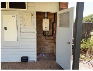
Line ID 131: Internal, Visiting Staff Rooms, Utilities Closets, SW Closet, Flue to The Domestic Hot Water System, Asbestos Containing Flue - Chrysotile & Amosite Asbestos Detected
