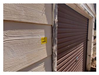
Line ID 134: External, Client Services Coordinator Residence, Garage, Elevations and Eaves Throughout, White Paint - Lead Detected (0.18% w/w)
