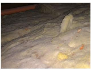
Line ID 165: Internal, Service Coordinator Residence, Ceiling Space Throughout, Floor Between Timber Framework, Insulation Batts - Suspected SMF
