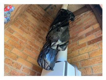
Line ID 80: Internal, Goonal and Mullion Lodge, Utilities Closets, NE And SW Closets, Flue to Hot Water System, Formed AC Flue - Chrysotile & Amosite Asbestos Detected
