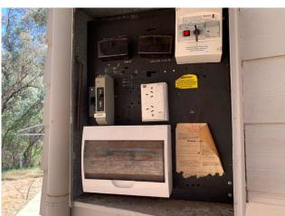
Line ID 20: External, Lakeside Cottages 1 & 2, Northwest Corner of Cottage 2 in Mounted Metal box, Bituminous Electrical Backing Board - Chrysotile Asbestos Detected
