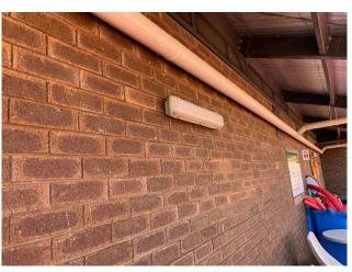
Line ID 189: Internal, Swimming Pool Complex, Pump House and Ablutions Building, Throughout, Single Long Tube Light Fittings, Capacitors - Suspected PCB
