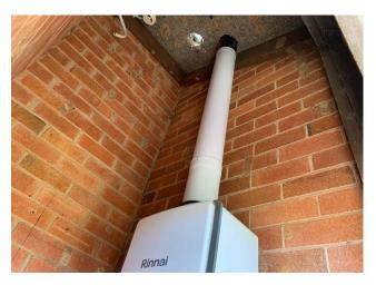
Line ID 112: Internal, Meroo and Yarraman Lodge, Utilities Closets, NE Closet, In Base Collar Of Hot Water System Flues, Woven Rope - Removed
