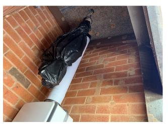
Line ID 116: Internal, Meroo and Yarraman Lodge, Utilities Closets, SW Closet, In Base Collar Of Hot Water System Flues, Woven Ripe - Suspected Asbestos
