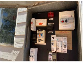
Line ID 40: External, Services Coordinator Residence, Elevations, Within Recessed Metal Box at The SE Corner of The Residence, Bituminous Electrical Backing Board - Chrysotile Asbestos Detected
