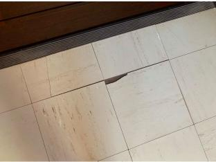
Line ID 67.2: Internal, Dining Hall Complex, Level 1 Throughout, Floor Covering, Vinyl Floor Tiles (Beige With Brown Fleck) - Chrysotile Asbestos Detected
