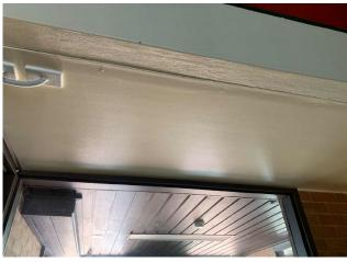
Line ID 53: Internal, Administration Complex, South Section Level 1, Balustrade, Thick Infill Panels, Compressed Cement Sheet - Chrysotile Asbestos Detected
