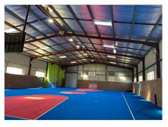
Line ID 164: Internal, Recreational Hall, Internal, Ceiling Space Throughout, Underside of Roof, Foil Backed Insulation Material - Suspected SMF
