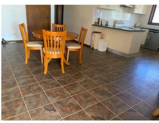
Line ID 121: Internal, Service Coordinator Residence, Kitchen, Floor Covering , Brown Flecked Vinyl Floor Tiles - Suspected Asbestos
