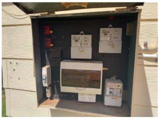
Line ID 9: External, Client Services Coordinator Residence, Residence, West Side , Bituminous Backing Board - Chrysotile Asbestos Detected
