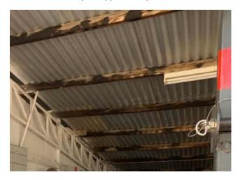
Line ID 186: Internal, Maintenance Workshop, Garage, Storage Room, Twin Long Tube Lights, Capacitor(s) -Suspected PCB
