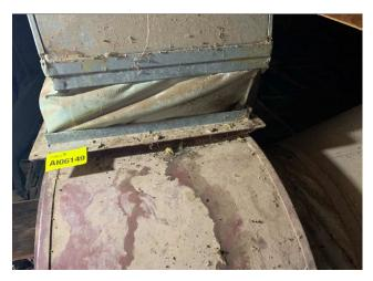
Line ID 68: Internal, Dining Hall Complex, Level 1, West Ceiling Space, Between Ductwork, Fabric Vibration Dampener - No Asbestos Detected
