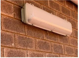
Line ID 181: Internal, Dining Hall Complex, Elevations, Wall Mounted Fittings Throughout, Representative Image Single Short Tube Light Fixtures, Capacitor(s) - PCB Capacitor
