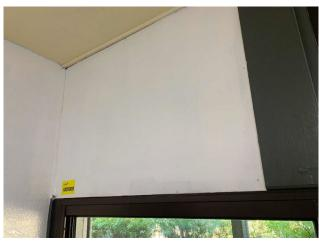
Line ID 65: Internal, Dining Hall Complex, Kitchen Store Rooms And Office, Office, Above West Entry, Panel, Compressed Cement Sheet - No Asbestos Detected
