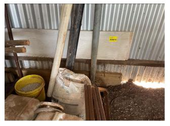
Line ID 100: Internal, Maintenance Workshop, Garage, North Storage Area, West Wall, Stored Planks on Wall, Profiled Fibre Cement Sheet Plank - Chrysotile Asbestos Detected
