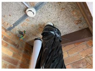
Line ID 128: Internal, Visiting Staff Rooms, Utilities Closets, NE Closet, Base Collar of Hot Water System Flues, Woven Rope Within Flue Pipe - Chrysotile Asbestos Detected
