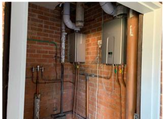
Line ID 156: Internal, Dining Hall Complex, West Hot Water Closet, Pipework, Insulation Material - Suspected SMF
