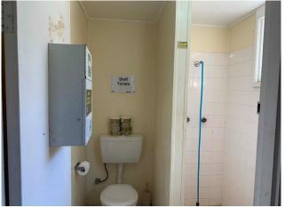
Line ID 103: Internal, Maintenance Workshop, Garage, Toilets and Store Room, Ceiling Lining and Joinery, Compressed Cement Sheet - Chrysotile Asbestos Detected
