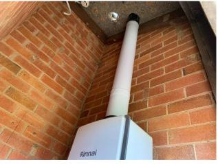
Line ID 111: Internal, Meroo and Yarraman Lodge, Utilities Closets, NE Closet, Formed AC Flue To The Domestic Hot Water System, Asbestos Containing Flue - Removed
