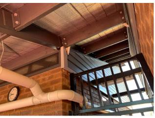
Line ID 168: Internal, Swimming Pool Complex, Pump House, Underside of Roof, Foil Backed Insulation Material - Suspected SMF
