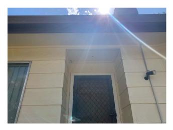
Line ID 11: External, General Managers Residence, East (Main) & West (Rear), Veranda Ceiling, Compressed Cement Sheet - Chrysotile Asbestos Detected
