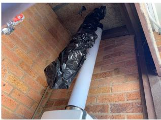
Line ID 80.1: Internal, Goonal and Mullion Lodge, Utilities Closets, NE And SW Closets, Flue to Hot Water System, Formed AC Flue - Chrysotile & Amosite Asbestos Detected
