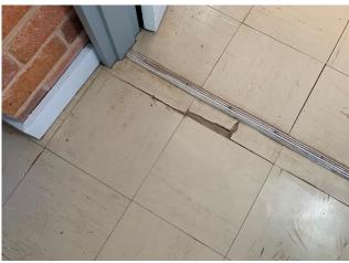
Line ID 67: Internal, Dining Hall Complex, Level 1 Throughout, Floor Covering, Vinyl Floor Tiles (Beige With Brown Fleck) -Chrysotile Asbestos Detected
