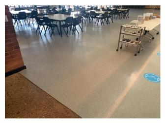
Line ID 62: Internal, Dining Hall Complex, Ground Level Dining Room And Middle Corridor, Below Linoleum Floor Covering, Beige With Brown Color Vinyl Floor Tiles - Chrysotile Asbestos Detected
