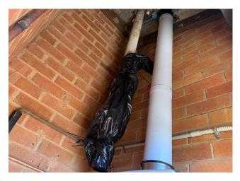
Line ID 129: Internal, Visiting Staff Rooms, Utilities Closets, NE Closet, Domestic Hot Water System, Flue Pipes - Chrysotile & Amosite Asbestos Detected
