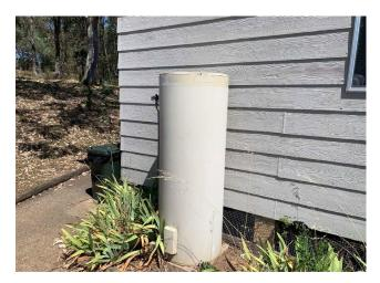
Line ID 141: External, Lakeside Cottages 1 & 2, Elevations, SW Corner, Rheem Domestic Hot Water System, Internal Insulation Material - Suspected SMF
