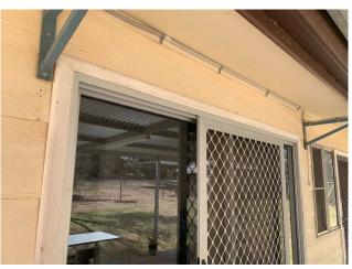
Line ID 12: External, General Managers Residence, Elevations, Perimeter of Residence, Eaves Lining, Compressed Cement Sheet - Chrysotile Asbestos Detected
