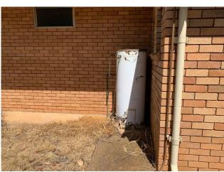
Line ID 142: External, Maintenance Workshop, Garage, West Side, Zip Domestic Hot Water System, Internal Insulation Material - Suspected SMF
