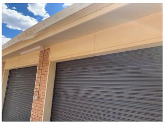
Line ID 29: External, Maintenance Workshop, Garage, East & West Elevations, Eaves Lining & Joinery, Compressed Cement Sheet - Chrysotile Asbestos Detected
