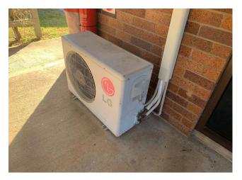
Line ID 209: External, Services Coordinator Residence, Elevations, West Elevation, Refrigerant Gas to the AC System, R22 Hydrochlorofluorocarbon (HCFC) - ODS Refrigerant
