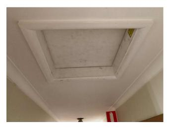
Line ID 120: Internal, Service Coordinator Residence, Garage, Ceiling, Manhole Cover, Compressed Cement Sheet - Chrysotile Asbestos Detected
