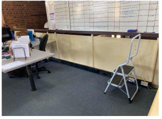
Line ID 49: Internal, Administration Complex, North Section, Balustrade Between Split Levels, Thick Infill Panels, Compressed Cement Sheet - Chrysotile Asbestos Detected
