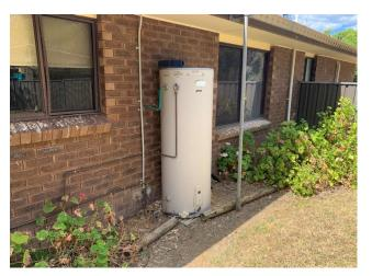
Line ID 143: External, Services Coordinator Residence, Elevations, North Side of Residence, Vulcan Domestic Hot Water System, Internal Insulation Material - Suspected SMF
