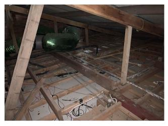
Line ID 153: Internal, Dining Hall Complex, Ceiling Space Above Dining Hall, Hot Water Pipe Work, Foil Wrapped Insulation Material - Suspected SMF
