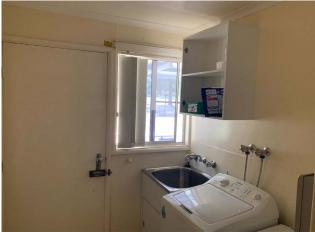
Line ID 56: Internal, Client Services Coordinator Residence, Laundry and Toilet, West Entry, Flat Wall Lining and Joinery, Compressed Cement Sheet - Chrysotile & Amosite Asbestos Detected
