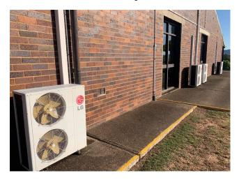
Line ID 194: External, Dining Hall Complex, South Side of Complex, Refrigerant Gas to The 'LG' AC Split System, R22 Hydrochlorofluorocarbon (HCFC) - ODS Refrigerant
