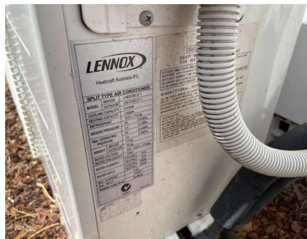
Line ID 60: External, Reception, Ground Floor, North-East Elevation, Air Conditioning Unit, R22 Hydrochlorofluorocarbon (HCFC) - ODS Refrigerant
