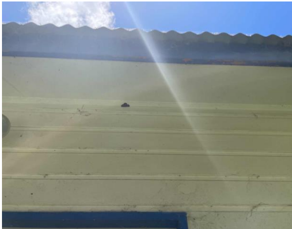
Line ID 3: External, Boat Maintenance Shed, Ground Floor, Eaves, Fibre Cement Sheeting - Suspected Asbestos
