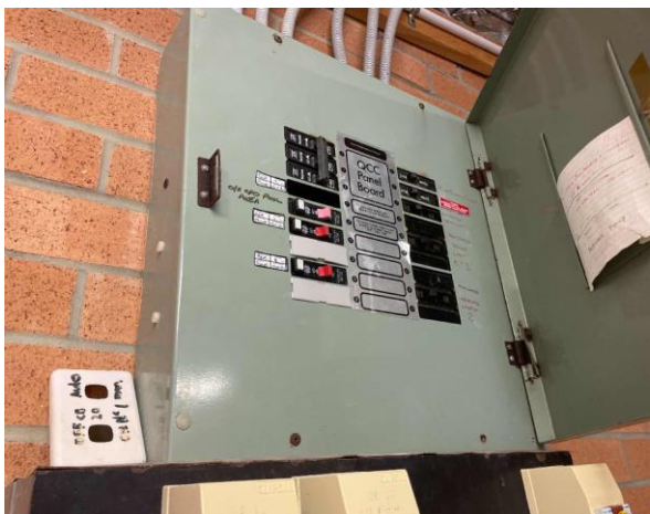
Line ID 29: Internal, Pool Pump and Storerooms, Ground Floor, Wall Mounted Cupboard, HRC Fuses - Suspected Asbestos
