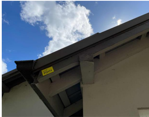
Line ID 34: External, Dining Room, Throughout, Gables, Brown Paint - Lead Detected ( 1.3\% w/w)
