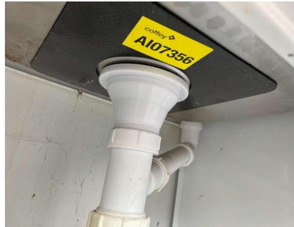
Line ID 26: Internal, Laundry, Ground Floor, Under Laundry Sinks, Sink Pad, Bituminous Membrane - No Asbestos Detected
