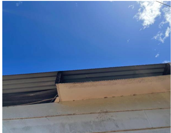
Line ID 9.1: External, Maintenance Shed, Ground Floor, Eaves to Shed and Debris From Damaged Eaves, Fibre Cement Sheetting - No Asbestos Detected
