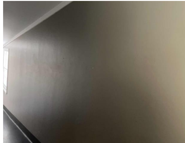
Line ID 44: Internal, Dining Room, Level 1, Adjacent Entrance and Corridor, Walls, Grey (Dark) Paint - Lead Detected (3.3% w/w)
