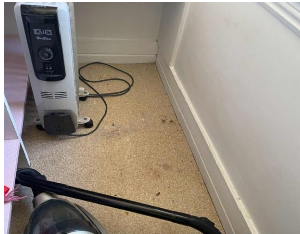
Line ID 32: Internal, Staff Residence, Ground Floor, Pantry Room, Vinyl Sheet - No Asbestos Detected
