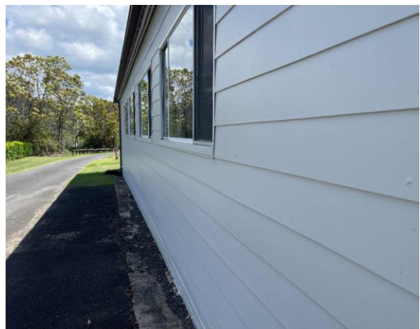
Line ID 12: External, Platypus Lodge, Ground Floor, Walls, Weatherboard Cladding, Fibre Cement Sheetting - No Asbestos Detected
