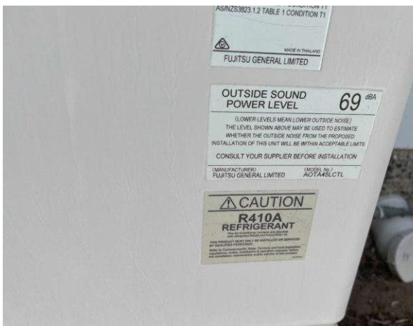
Line ID 59: External, Platypus Lodge, Ground Floor, West Elevation, Air Conditioning Unit, R410A Hydrofluorocarbon (HFC) - Non ODS Refrigerant
