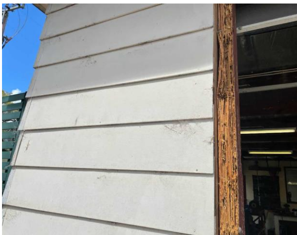
Line ID 11: External, Maintenance Shed, Ground Floor, Walls, Weatherboard Cladding, Fibre Cement Sheetting - No Asbestos Detected
