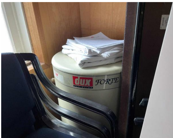
Line ID 53: Internal, Conference Room, Ground Floor, Conference Storeroom, Hot Water Heater, Insulation Material - Suspected SMF
