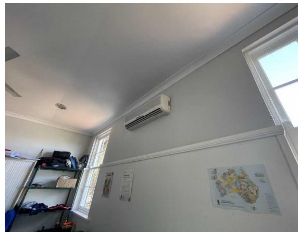
Line ID 64: Internal, Conference Room, Ground Floor, South Elevation, Air Conditioning Unit, Unknown Refrigerant - Suspected ODS
