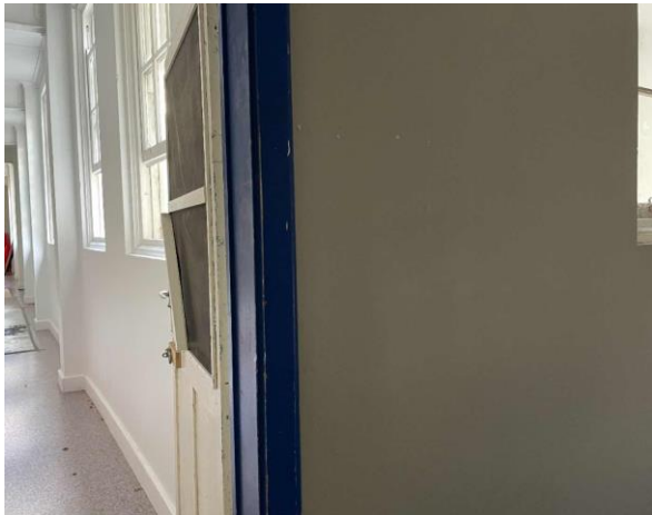
Line ID 43: Internal, Dining Room, Ground Level, Lower Area Entrance, Door Frame, Blue (Dark) Paint - Lead Detected (0.051% w/w)
