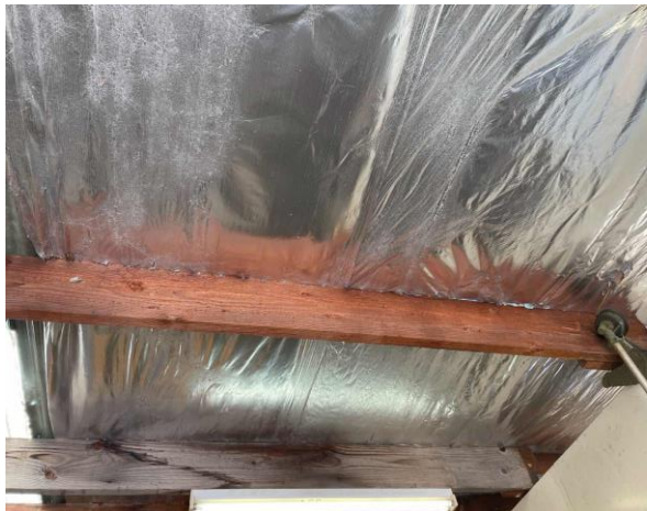
Line ID 49: External, Maintenance Shed, Ground Floor, Underside of Roof, Sarking Insulation - Suspected SMF
