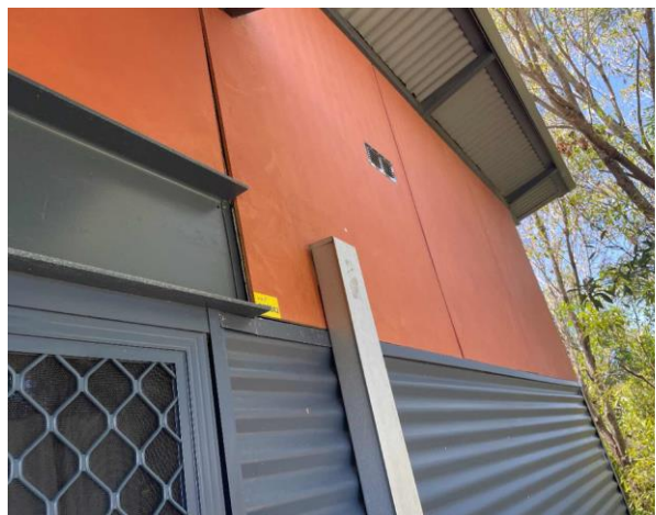
Line ID 18: External, Units 1-5, Ground Floor, Upper Wall Lining, Compressed Cement Sheet - No Asbestos Detected
