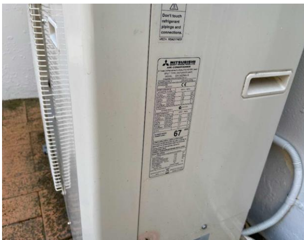
Line ID 65: Internal, Conference Room, Ground Floor, West Elevation, Air Conditioning Unit, R410A Hydrofluorocarbon (HFC) - Non ODS Refrigerant
