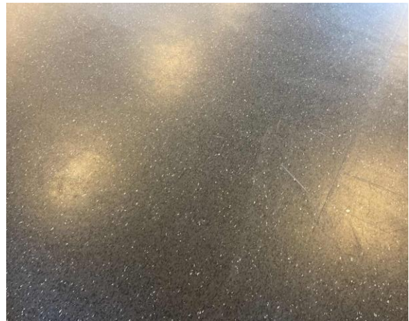
Line ID 22: Internal, Dining Room, Ground Level, Throughout Dining Hall and Bathrooms, Floor Covering, Black Speckled Vinyl Sheet - No Asbestos Detected
