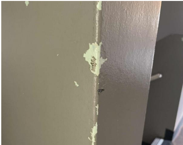
Line ID 45: Internal, Dining Room, Level 1, s Adjacent Entrance and Corridor, Lower Layer Paint to Wall, Cream Paint - Lead Detected (2.3% w/w)
