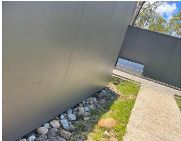
Line ID 16: External, Recreation Hall, Ground Floor, Wall Lining, Compressed Cement Sheet - No Asbestos Detected
