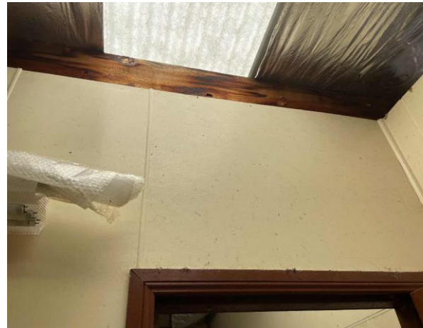
Line ID 28: Internal, Maintenance Shed, Ground Floor, Storage Room, Wall Lining, Compressed Cement Sheetting - No Asbestos Detected
