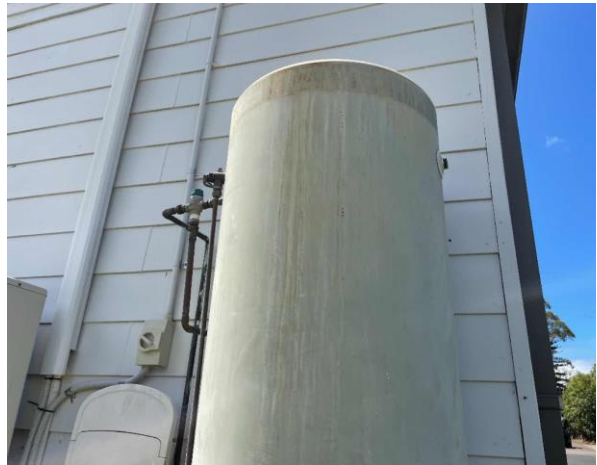
Line ID 50: External, Platypus Lodge, Ground Floor, West Elevation, Hot Water Heater, Insulation Material - Suspected SMF
