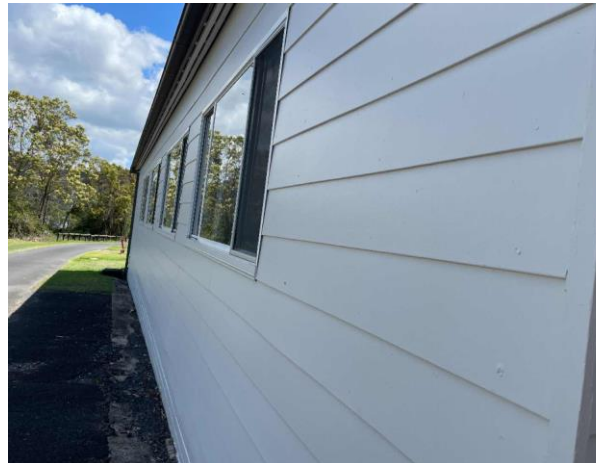
Line ID 38: External, Platypus Lodge, Ground Floor, Walls, White Paint - Lead Detected (<0.005% w/w)
