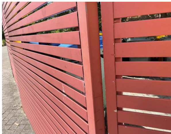
Line ID 36: External, Garbage and Fire Pump Rooms, Ground Floor, Garbage Bins Fence, Red Paint - Lead Detected ( <0.005\% w/w)
