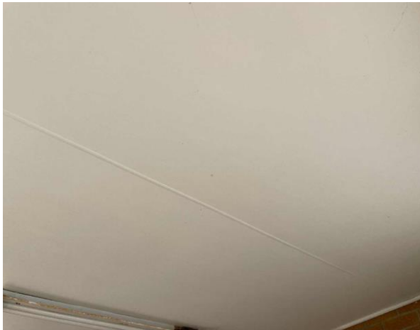
Line ID 13: External, Pool Area, Ground Floor, Ceiling Lining Adjacent Entrance to Pool Pump Room, Compressed Cement Sheeting - No Asbestos Detected
