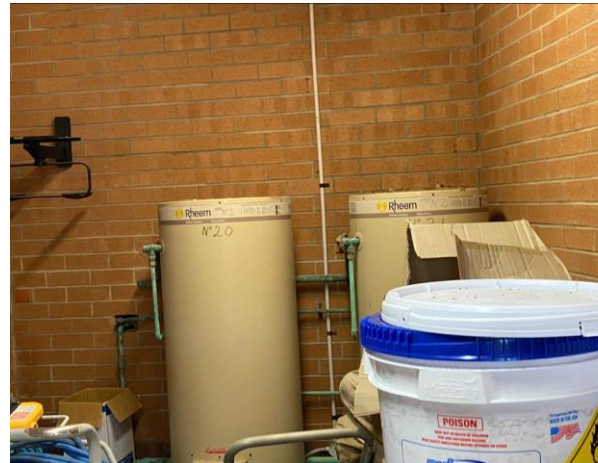
Line ID 56: Internal, Pool Pump and Storerooms, Ground Floor, Within Storeroom, Hot Water Heater, Insulation Material - Suspected SMF
