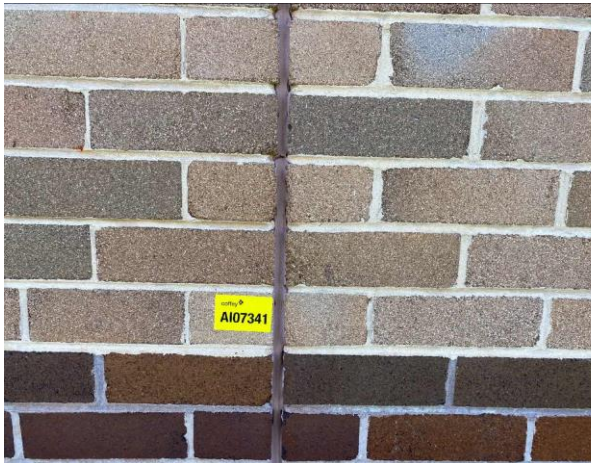
Line ID 1: External, Accommodation Lodges, Lorikeet, Kookaburra, Waratah, Koala and Possum, Throughout, Joint Mastic Between Bricks, Construction Joint Mastic - No Asbestos Detected
