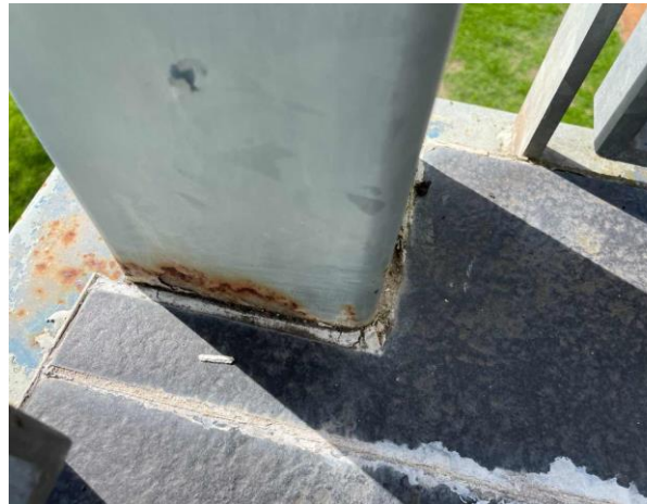
Line ID 4: External, Dining Room, Throughout, East Side Dining Area, Poles to Ground, Mastic Sealant - No Asbestos Detected
