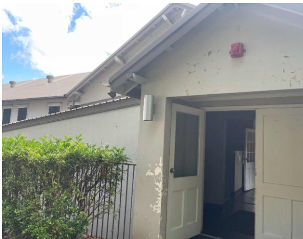
Line ID 35: External, Dining Room, Throughout, Walls, Grey (Light) Paint - Lead Detected ( 15\% w/w)
