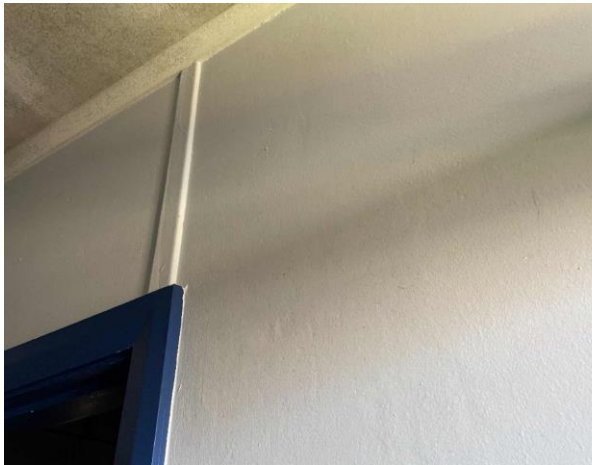
Line ID 31: Internal, Reception, Ground Floor, Store and Redundant Bathroom Walls, Corrugated Cement Sheet - Chrysotile, Amosite and Crocidolite Asbestos Detected
