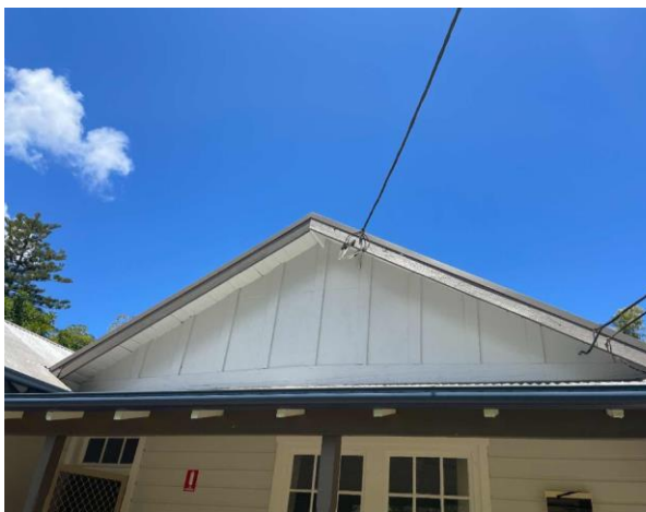
Line ID 17: External, Staff Residence, Ground Floor, Fascia Panels to Gable, Fibre Cement Sheeting - Suspected Asbestos
