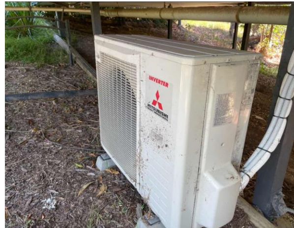
Line ID 62: External, Units 1-5, Ground Floor, Air Conditioning Unit, R410A Hydrofluorocarbon (HFC) - Non ODS Refrigerant
