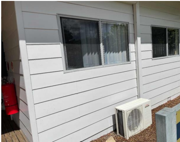
Line ID 15: External, Reception, Ground Floor, Walls, Weatherboard Cladding, Fibre Cement Sheeting - No Asbestos Detected
