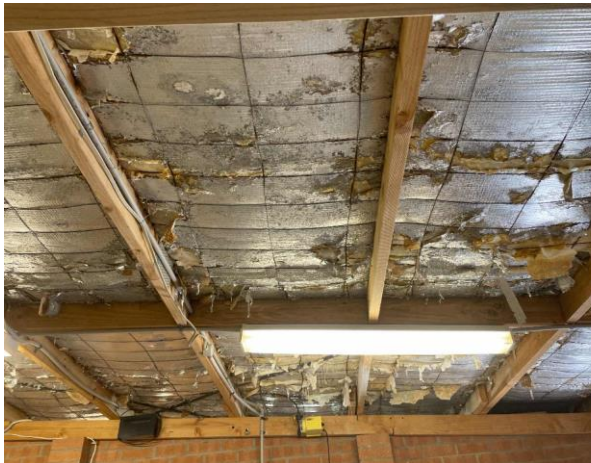
Line ID 55: Internal, Pool Pump and Storerooms, Ground Floor, Underside of Roof, Sarking Insulation - Suspected SMF
