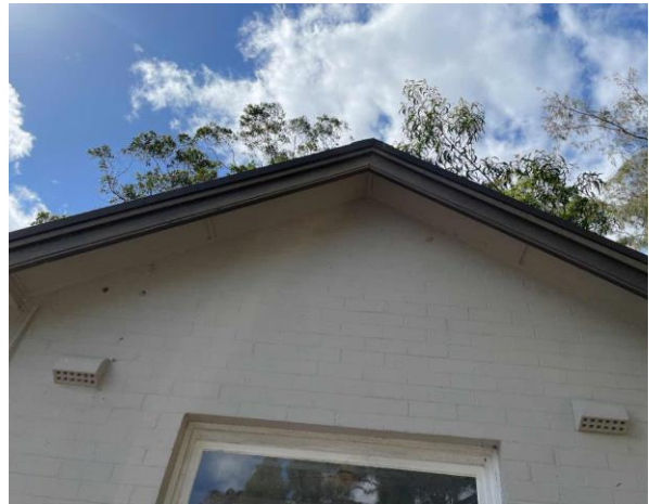
Line ID 8: External, Laundry, Ground Floor, Throughout Building, Eaves, Fibre Cement Sheetting - Suspected Asbestos
