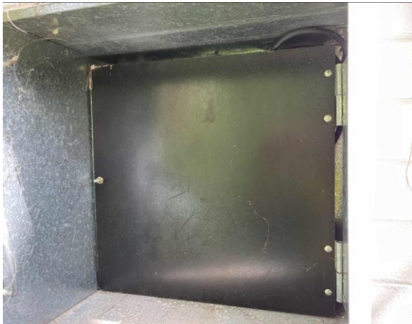
Line ID 27: Internal, Laundry, Ground Floor, Wall Mounted Cupboard, Electrical Board, Bituminous Backing Board - Suspected Asbestos
