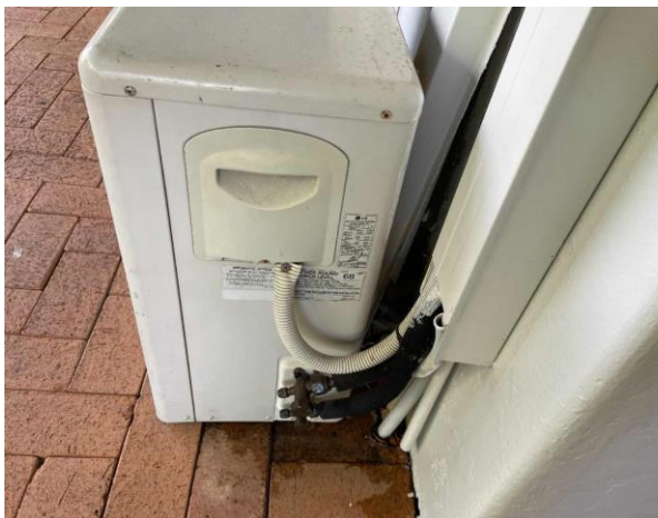
Line ID 63: Internal, Conference Room, Ground Floor, East Elevation, Air Conditioning Unit, R22 Hydrochlorofluorocarbon (HCFC) - ODS Refrigerant
