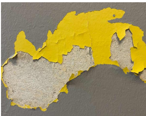
Line ID 41: Internal, Dining Room, Ground Level, Adjacent Entrance to Craft Area, Lower Layer Paint, Yellow Paint - Lead Detected (0.60% w/w)
