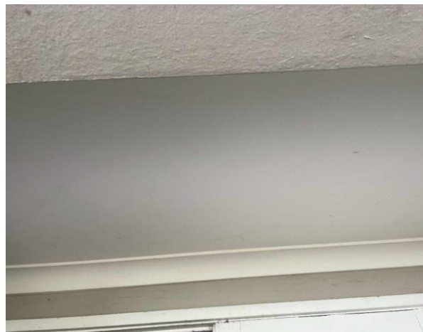
Line ID 6: External, Dining Room, Throughout, West Entrance Awning, Plaster Board - No Asbestos Suspected
