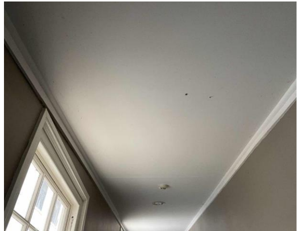
Line ID 20: Internal, Dining Room, Ground Level, Hallway Ramp, Ceiling, Compressed Cement Sheetting - Suspected Asbestos
