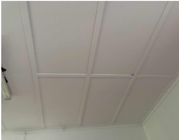
Line ID 21: Internal, Dining Room, Ground Level, Lower Area Ceiling, Compressed Cement Sheetting - Suspected Asbestos
