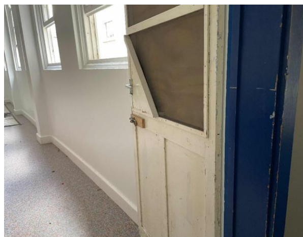
Line ID 42: Internal, Dining Room, Ground Level, Lower Area Entrance Door, White Paint - Lead Detected (0.006% w/w)
