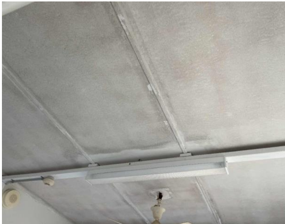
Line ID 25: Internal, Laundry, Ground Floor, to Ceiling Panels, Compressed Cement Sheetting - Suspected Asbestos
