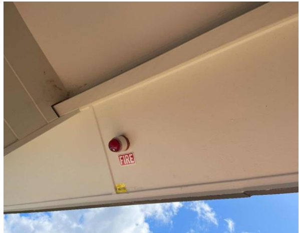
Line ID 14: External, Reception, Ground Floor, Eaves, Fibre Cement Sheeting - Chrysotile, Amosite and Crocidolite Asbestos Detected
