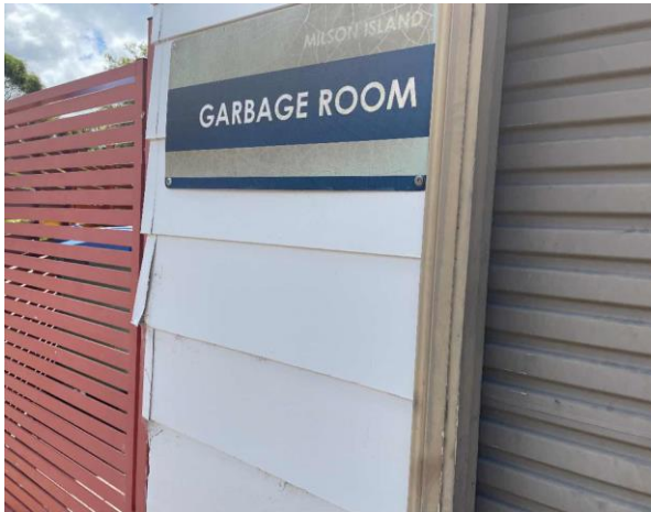
Line ID 7: External, Garbage and Fire Pump Rooms, Ground Floor, Garbage Room, Wall Lining, Fibre Cement Sheetting - No Asbestos Detected
