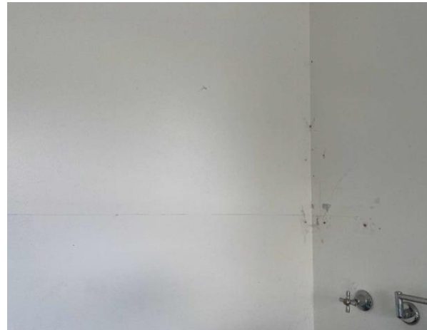
Line ID 46: Internal, Laundry, Ground Floor, Walls, White Paint - Lead Detected (<0.005% w/w)
