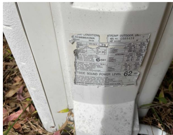
Line ID 66: Internal, Laundry, Ground Floor, South Elevation, Air Conditioning Unit, R410A Hydrofluorocarbon (HFC) - Non ODS Refrigerant
