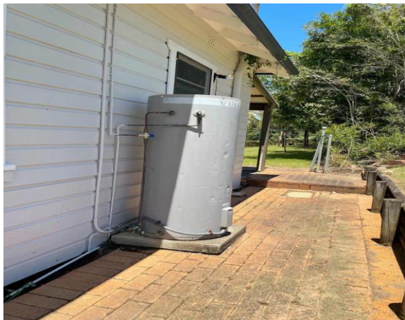
Line ID 51: External, Staff Residence, Ground Floor, West Elevation, Hot Water Heater, Insulation Material - Suspected SMF
