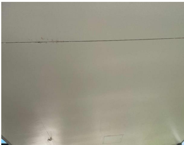
Line ID 5: External, Dining Room, Throughout, East Side Dining Area, Underside of Canopy, Compressed Cement Sheeting - Suspected Asbestos
