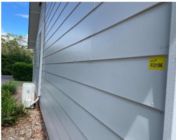
Line ID 39: External, Reception, Ground Floor, Walls, White Paint - Lead Detected (<0.005% w/w)
