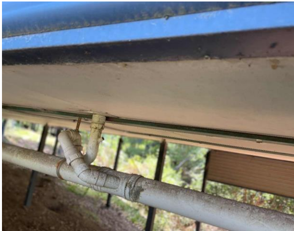
Line ID 19: External, Units 1-5, Ground Floor, Waterproofing Membrane to Underside of Unit, Fibre Cement Sheetting - No Asbestos Detected
