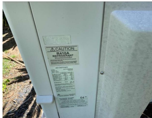
Line ID 58: External, Accommodation Lodges, Lorikeet, Kookaburra, Waratah, Koala and Possum, Air Conditioning Unit, R410A Hydrofluorocarbon (HFC) - Non ODS Refrigerant
