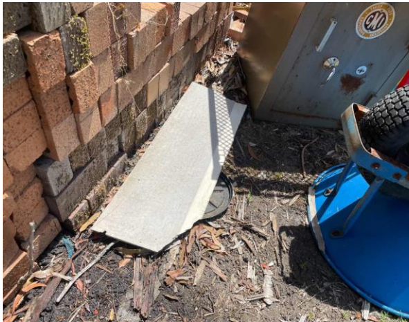
Line ID 9: External, Maintenance Shed, Ground Floor, Eaves to Shed and Debris From Damaged Eaves, Fibre Cement Sheetting - No Asbestos Detected
