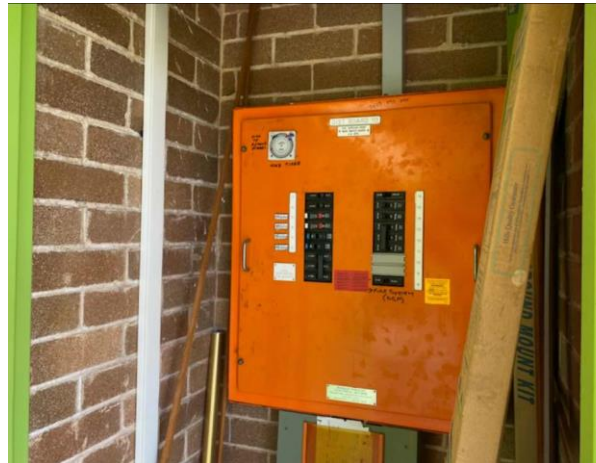
Line ID 2: External, Accommodation Lodges, Lorikeet, Kookaburra, Waratah, Koala and Possum, Wall Mounted Electrical Cupboards, HRC Fuses - Suspected Asbestos
