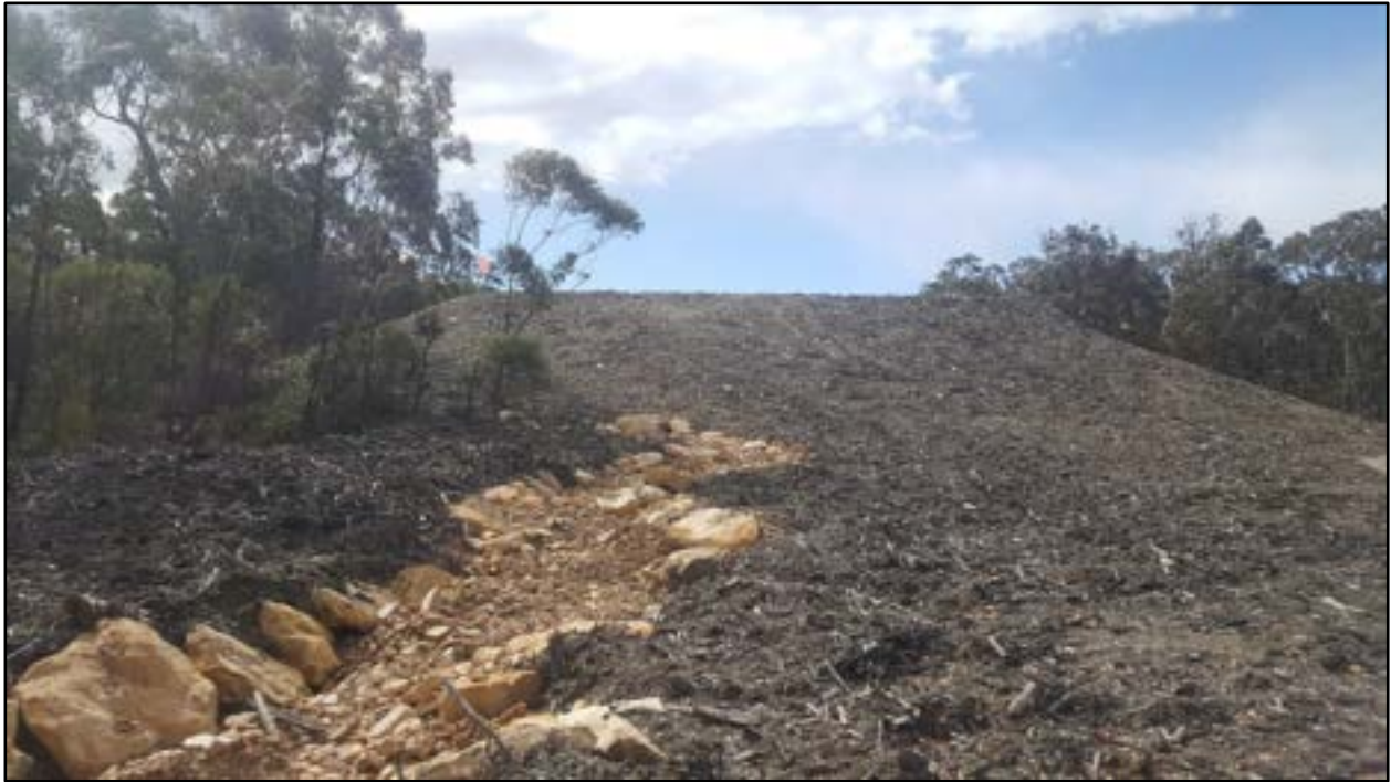
Plate 10b. The disturbed area at the southern end of the 800 m rifle range. Note the attempted rehabilitation measures of mulching and rock placement (date taken: 08/08/19).
