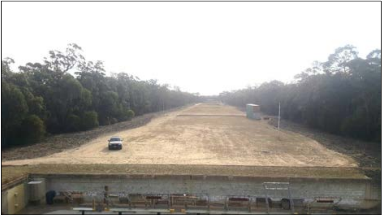
Plate 10a. Looking north-east along existing 800 m rifle range (date taken: 08/09/2019).
