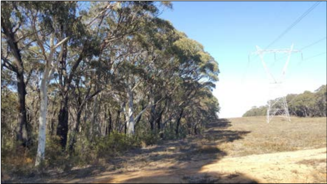
Plate 9c. Looking south-west with the conservation area evident to the west of the powerline easement (right of photograph) (date taken: 30/8/2018).
