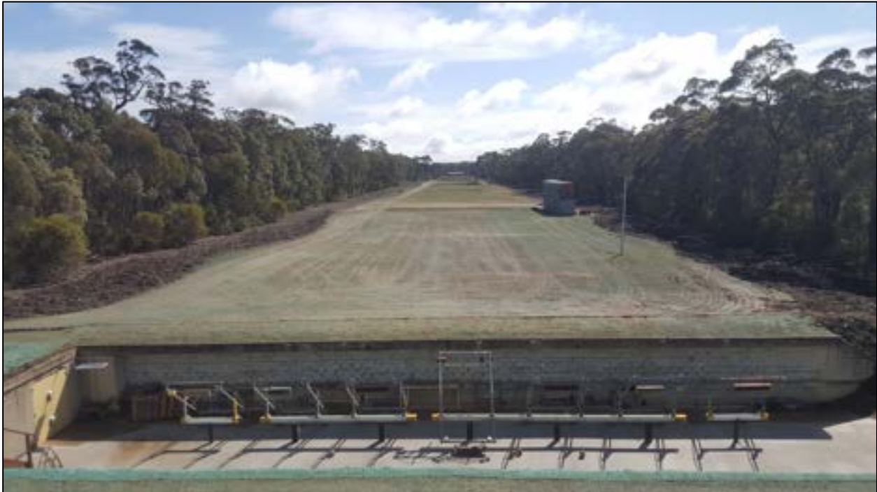
Plate 10a. Looking north-east along existing 800 m rifle range (date taken: 18/10/2018).
