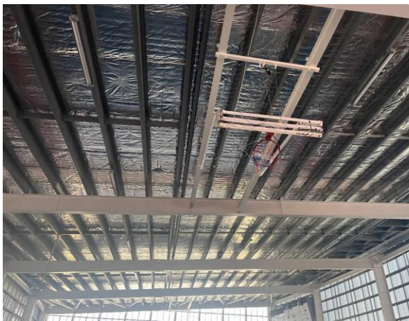
Line ID 55: Internal, Stadium, Gym, Underside of Roof, Sarking Insulation - Suspected SMF
