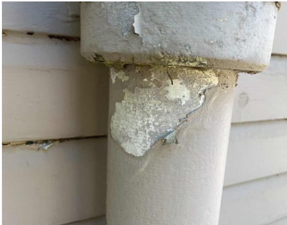
Line ID 23: External, Toilets to the North of Murph's Cottages, Entrance and Surrounds, Rear of Female Toilet, Down Pipe, Moulded Fibre Cement - Chrysotile and Amosite Asbestos Detected
