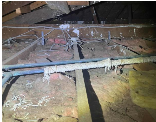
Line ID 27: Internal, Centre Managers House, Laundry, Pipework, Rope Insulation, Woven Material - Chrysotile Asbestos Detected
