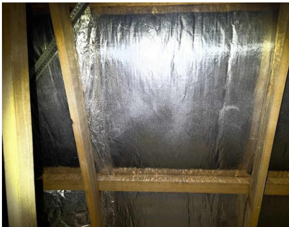
Line ID 53: Internal, Reception, Ceiling Void, Underside of Roof, Sarking Insulation - Suspected SMF
