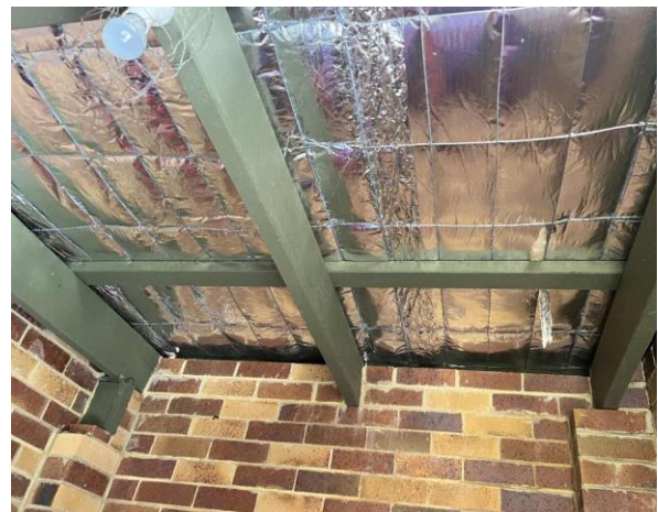
Line ID 56: Internal, Swimming Pool Change and Toilets, Free Play Ports Store, Underside of Roof, Sarking Insulation - Suspected SMF
