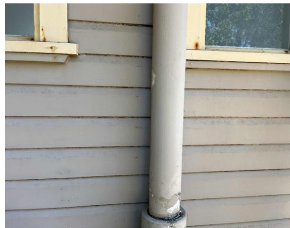
Line ID 45: External, Toilets to the North of Murph's Cottages, Entrance and Surrounds, Down Pipe and Walls, Beige Paint - Lead Detected (0.18% w/w)
