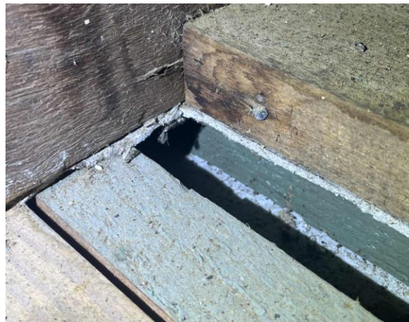
Line ID 28: Internal, Centre Managers House, Laundry, Second Skin Ceiling Lining, Fibre Cement Sheet - Chrysotile Asbestos Detected
