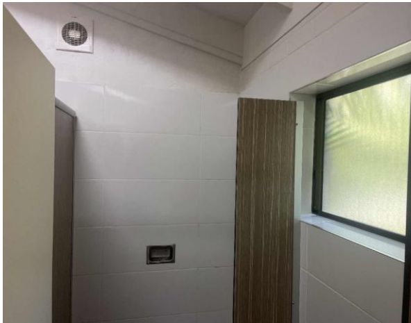
Line ID 29: Internal, Lodge 14, Toilet, Behind Ceramic Tiles to Walls, Fibre Cement Sheet - Chrysotile Asbestos Detected
