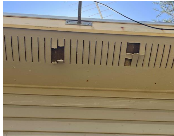
Line ID 12.1: External, Murphy's Cottage Block, Veranda and Undercover Area, Debris to the Floor From the Eave to Rear of Kitchen, Fibre Cement Debris - Chrysotile Asbestos Detected
