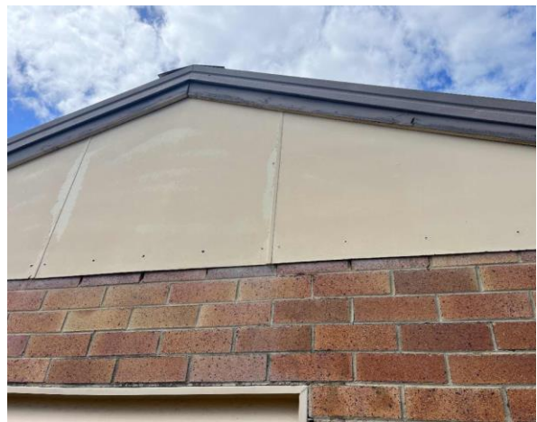
Line ID 19: External, Swimming Pool Toilets and Change, Swimming Pool Plant Room, Infill Panels above Walls, Fibre Cement Sheet - No Asbestos Detected
