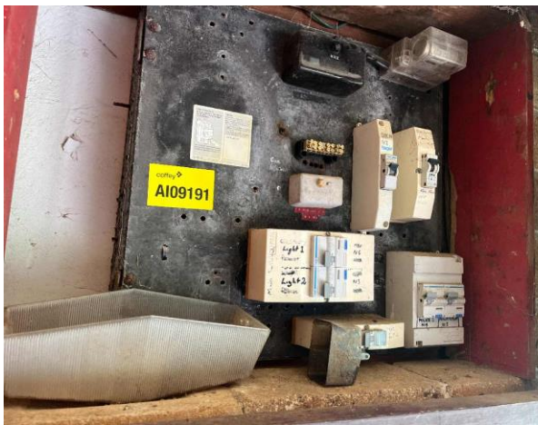
Line ID 17: External, Services Coordinator Residence, Entry And Covered Walkways, Electrical Box adjacent Entry, Bituminous Backing Board - Chrysotile Asbestos Detected
