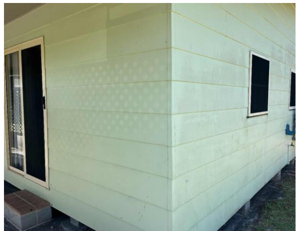
Line ID 4: External, Beachside Lodge, Veranda and Walls, Weatherboard Wall Lining, Fibre Cement Sheet - No Asbestos Detected
