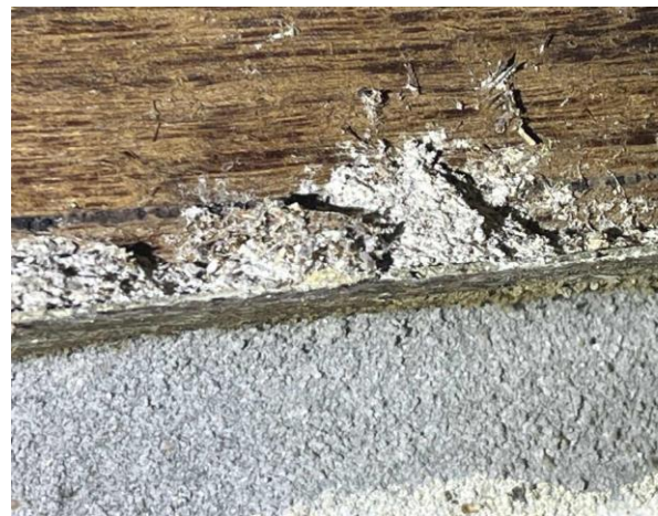
Line ID 26: Internal, Centre Managers House, Garage, Timber Beams, Fibre Cement Sheet Debris - Chrysotile Asbestos Detected
