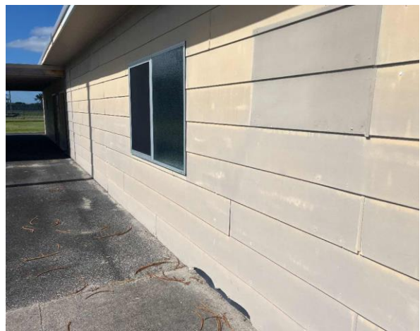
Line ID 9: External, Gym Shed, Entrance and Covered Walkway, Wall Lining, Fibre Cement Sheet - No Asbestos Detected
