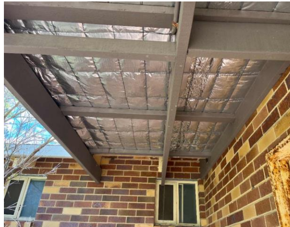
Line ID 49: External, Swimming Pool Toilets and Change, Free Play Sports Store, Roof Adjacent the Entry, Sarking Insulation - Suspected SMF
