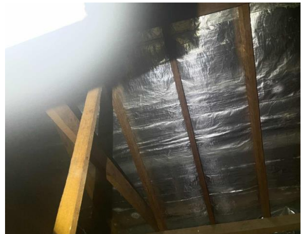
Line ID 54: Internal, Service Coordinator Residence, Ceiling Void, Underside of Roof, Sarking Insulation - Suspected SMF
