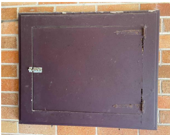
Line ID 44: External, Services Coordinator Residence, Entry And Covered Walkways, Electrical Box Adjacent Entry, Purple Paint - Lead Detected (0.18% w/w)
