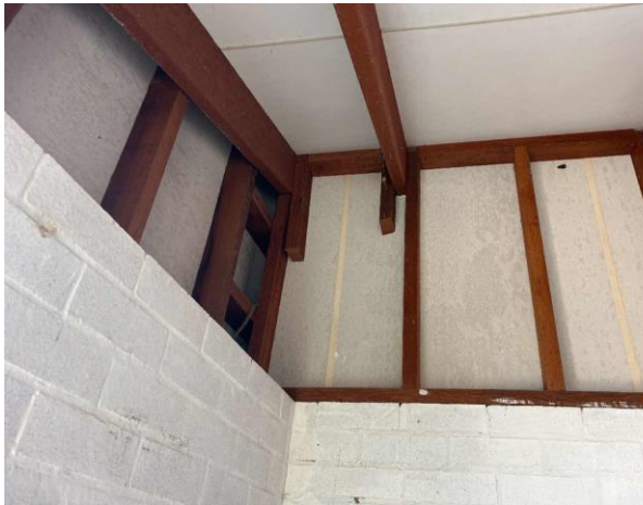
Line ID 35: Internal, Swimming Pool Change and Toilets, Storeroom Adjacent Female Change, Wall Linings, Fibre Cement Sheet - No Asbestos Detected
