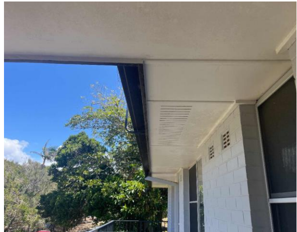
Line ID 6: External, Centre Managers Residence, Veranda, Eave Linings, Fibre Cement Sheet - Chrysotile Asbestos Detected
