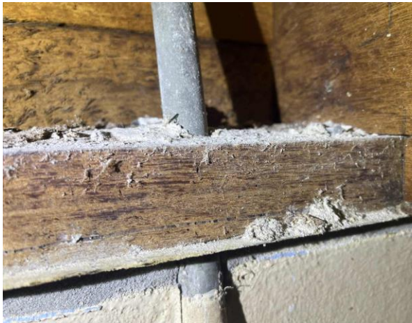
Line ID 26.3: Internal, Centre Managers House, Garage, Timber Beams, Fibre Cement Sheet Debris - Chrysotile Asbestos Detected
