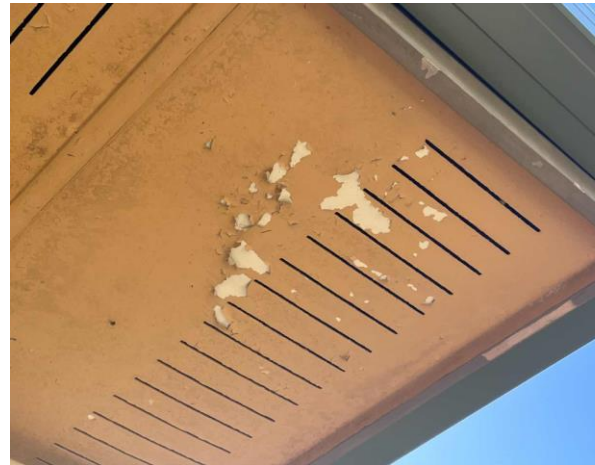
Line ID 42: External, Project Coordinators Residence, Entrance Area and Surrounds, Eave Linings, Beige Paint - Lead Detected (0.16% w/w)
