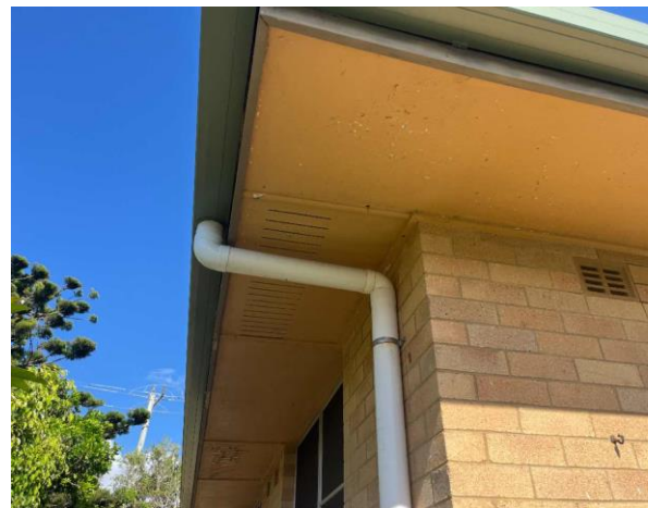
Line ID 14: External, Project Coordinators Residence, Entrance Area and Surrounds, Eave Linings, Fibre Cement Sheet - Chrysotile Asbestos Detected
