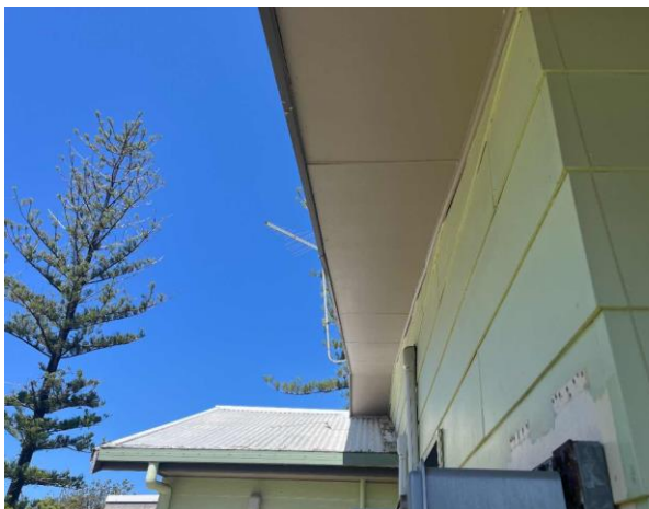
Line ID 3.1: External, Beachside Lodge, Veranda and Walls, Eaves, Fibre Cement Sheet - No Asbestos Detected
