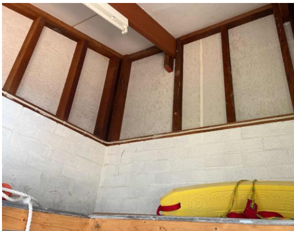
Line ID 37: Internal, Swimming Pool Change and Toilets, Storeroom Adjacent Male Toilets, Wall Linings, Fibre Cement Sheet - No Asbestos Detected
