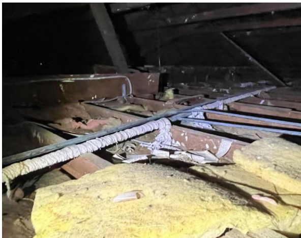
Line ID 27.1: Internal, Centre Managers House, Laundry, Pipework, Rope Insulation, Woven Material - Chrysotile Asbestos Detected
