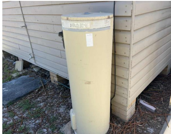
Line ID 47: External, Murphy's Cottage Block, Veranda and Undercover Area, Hot Water Unit, Insulation Material - Suspected SMF
