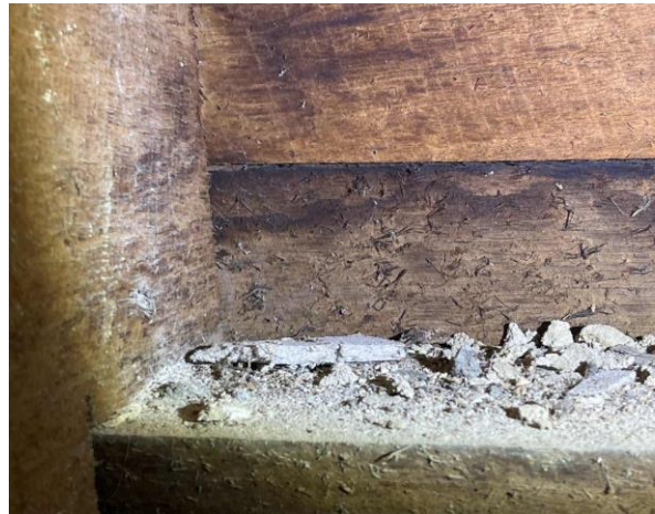
Line ID 26.2: Internal, Centre Managers House, Garage, Timber Beams, Fibre Cement Sheet Debris - Chrysotile Asbestos Detected
