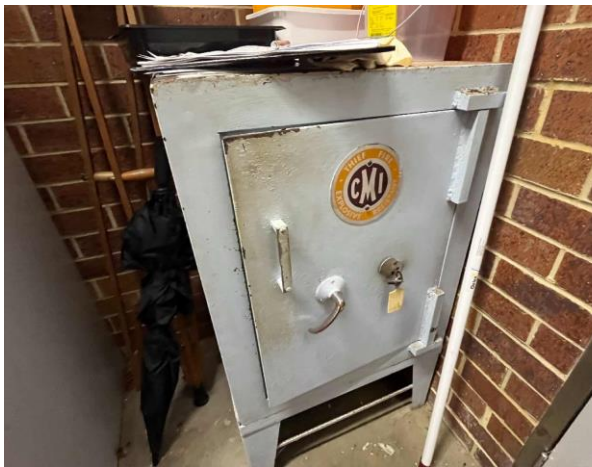
Line ID 33: Internal, Reception, Storeroom, Safe, Internal Insulation - Suspected Asbestos
