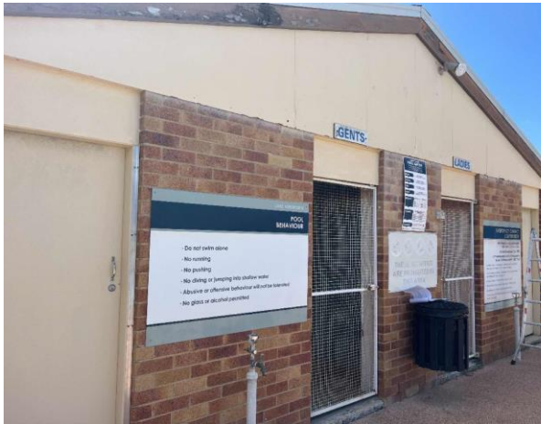
Line ID 21: External, Swimming Pool, Toilet Entry Area, Infill Panels Above Doors, Fibre Cement Sheet - Chrysotile and Amosite Asbestos Detected
