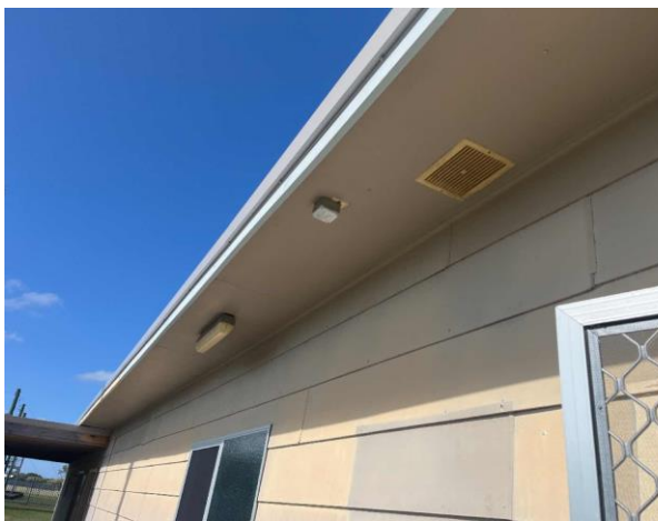
Line ID 8: External, Gym Shed, Entrance and Covered Walkway, Eaves, Fibre Cement Sheet - Chrysotile & Amosite Asbestos Detected
