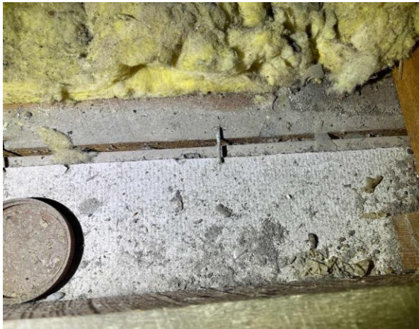
Line ID 31: Internal, Program Coordinator Residence, Laundry, Ceiling Lining, Fibre Cement Sheet - Chrysotile and Amosite Asbestos Detected
