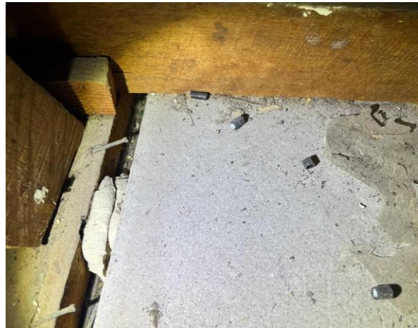
Line ID 32: Internal, Program Coordinator Residence, Laundry and Shower, Wall Lining, Fibre Cement Sheet - Chrysotile Asbestos Detected
