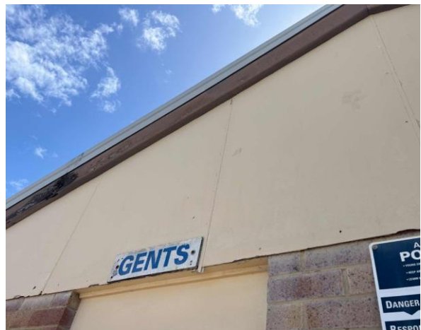
Line ID 20: External, Swimming Pool Toilets and Change, Toilet Entry Area, High Level Infill Panels Fascia, Fibre Cement Sheet - No Asbestos Detected
