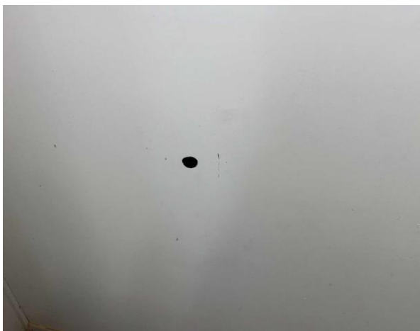
Line ID 39: Internal, Toilets North of Murph's Cottages, Throughout, Wall Lining, Fibre Cement Sheet - No Asbestos Detected
