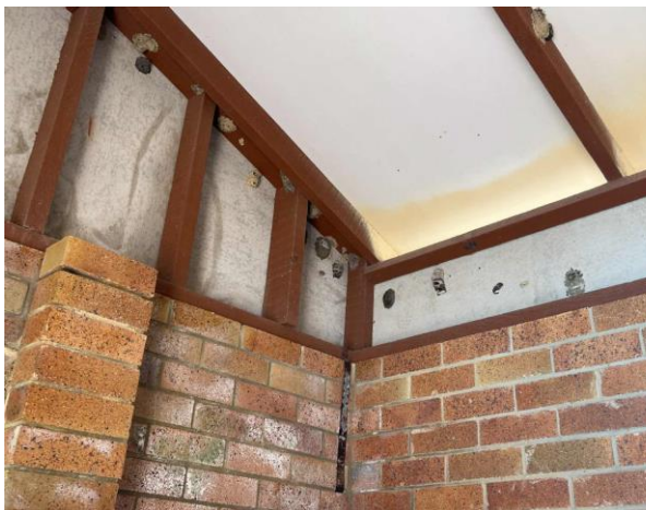
Line ID 19.1: External, Swimming Pool Plant Room, Infill Panels above Walls, Fibre Cement Sheet - No Asbestos Detected
