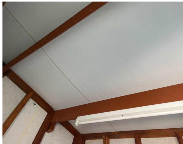
Line ID 34: Internal, Swimming Pool Change and Toilets, Storeroom Adjacent Female Change, Ceiling Linings, Fibre Cement Sheet - No Asbestos Detected
