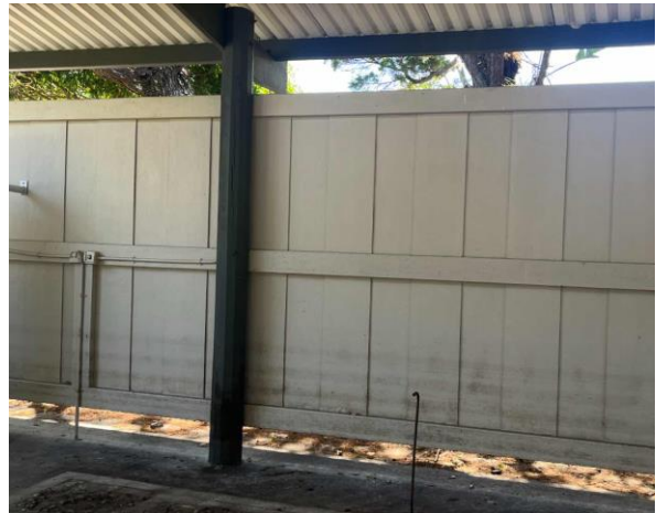
Line ID 2: External, BBQ Area, Throughout, Wall Lining, Fibre Cement Sheet - No Asbestos Detected
