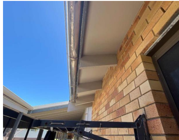
Line ID 11.1: External, Lodge 14, Covered Walkway, Eaves, Fibre Cement Sheet - Chrysotile Asbestos Detected
