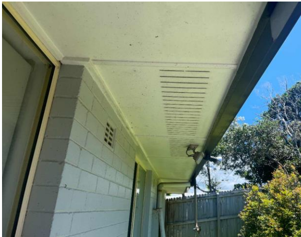
Line ID 6.1: External, Centre Managers Residence, Veranda, Eave Linings, Fibre Cement Sheet - Chrysotile Asbestos Detected
