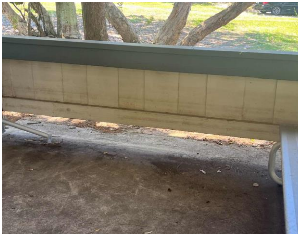
Line ID 2.1: External, BBQ Area, Throughout, Wall Lining, Fibre Cement Sheet - No Asbestos Detected
