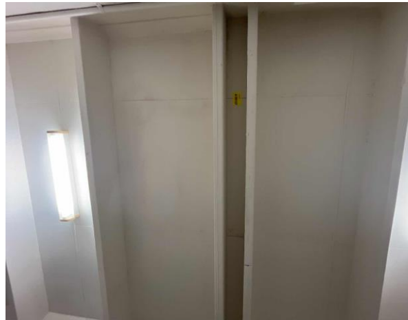
Line ID 30: Internal, Lodge 14, Toilet, Ceiling Lining, Fibre Cement Sheet - No Asbestos Detected
