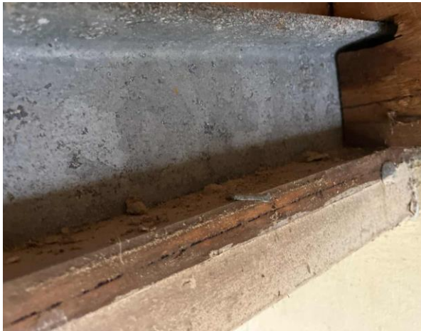
Line ID 26.1: Internal, Centre Managers House, Garage, Timber Beams, Fibre Cement Sheet Debris - Chrysotile Asbestos Detected
