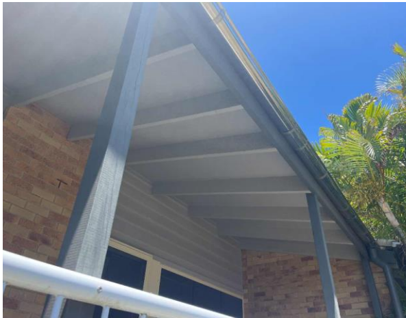
Line ID 11: External, Lodge 14, Covered Walkway, Eaves, Fibre Cement Sheet - Chrysotile Asbestos Detected
