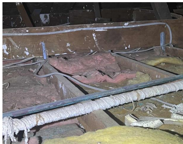
Line ID 50.1: Internal, Centre Managers House, Laundry, Throughout Ceiling Void, Insulation Batts - Suspected SMF
