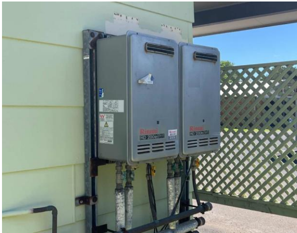
Line ID 46: External, Beachside Lodge, Veranda and Walls, Hot Water Units, Insulation Material - Suspected SMF
