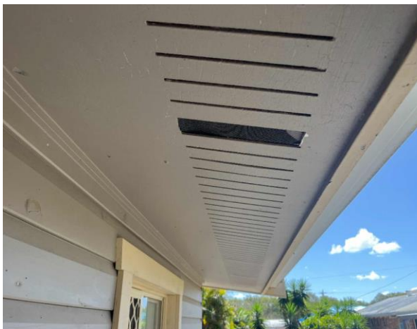
Line ID 13: External, Murphy's Cottage Block, Veranda and Undercover Area, Eave Linings, Fibre Cement Sheet - Chrysotile & Amosite Asbestos Detected
