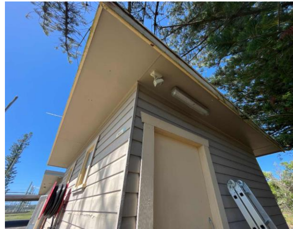
Line ID 22: External, Toilets to the North of Murph's Cottages, Entrance and Surrounds, Eaves, Fibre Cement Sheet - Chrysotile & Amosite Asbestos Detected
