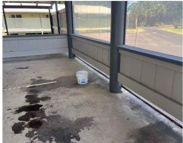
Line ID 7: External, Craft Area, Storage Shed, Wall Lining, Fibre Cement Sheet - No Asbestos Detected
