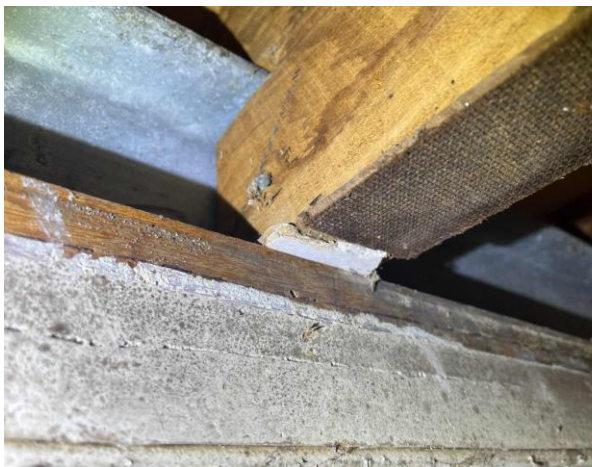
Line ID 25: Internal, Centre Managers House, Garage, Ceiling Space, Packer to Timber, Fibre Cement Sheet - Chrysotile and Amosite Asbestos Detected
