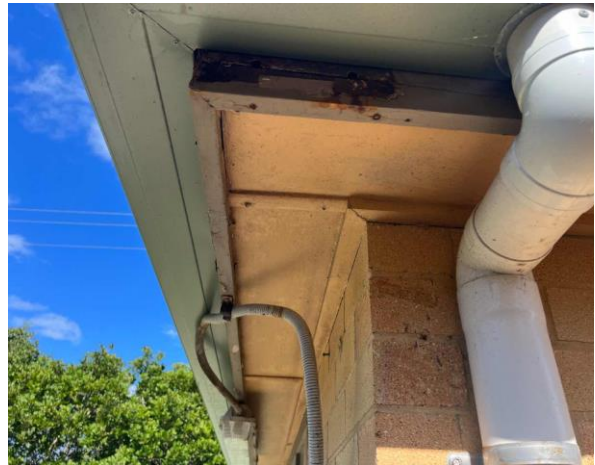
Line ID 16: External, Project Coordinators Residence, Rear Garage, Eaves, Fibre Cement Sheet - Chrysotile Asbestos Detected
