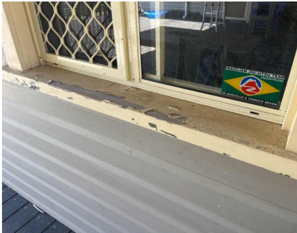
Line ID 41: External, Murphy's Cottage Block, Veranda and Undercover Area, Timber Window Frames, Cream Paint - Lead Detected (0.066% w/w)
