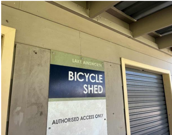
Line ID 5: External, Bike Store, Veranda, Wall Lining, Fibre Cement Sheet - No Asbestos Detected
