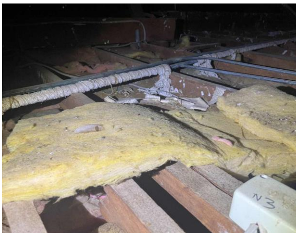
Line ID 50: Internal, Centre Managers House, Laundry, Throughout Ceiling Void, Insulation Batts - Suspected SMF
