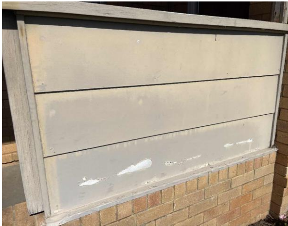
Line ID 15: External, Project Coordinators Residence, Entrance Area, Wall Lining and Entrance Sheeting, Fibre Cement Sheet - No Asbestos Detected
