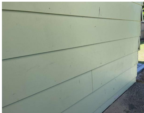
Line ID 40: External, Beachside Lodge, Veranda, Walls, Light Green Paint - Lead Detected (<0.005% w/w)
