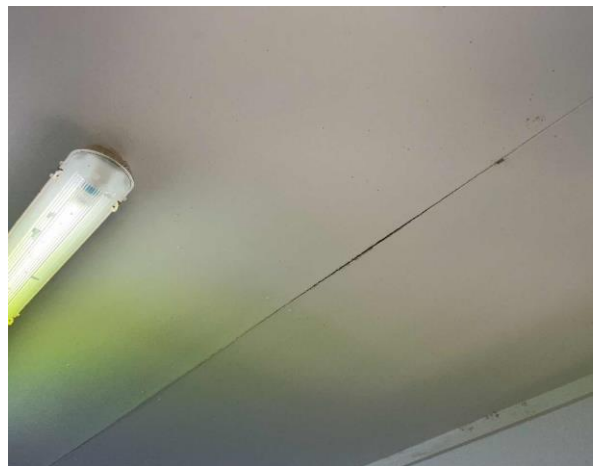
Line ID 38: Internal, Toilets North of Murph's Cottages, Throughout, Ceiling, Fibre Cement Sheet - No Asbestos Detected
