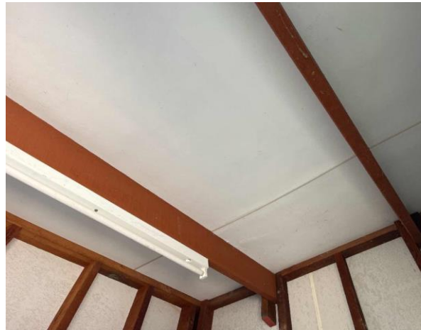
Line ID 36: Internal, Swimming Pool Change and Toilets, Storeroom Adjacent Male Toilets, Ceiling Linings, Fibre Cement Sheet - No Asbestos Detected
