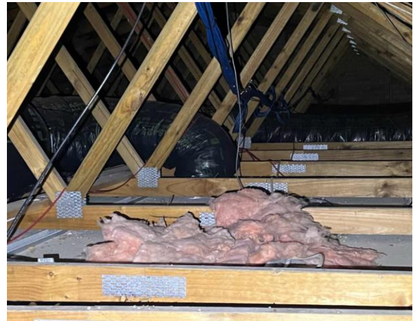
Line ID 52: Internal, Reception, Ceiling Void, Loose Insulation, Insulation Batts - Suspected SMF
