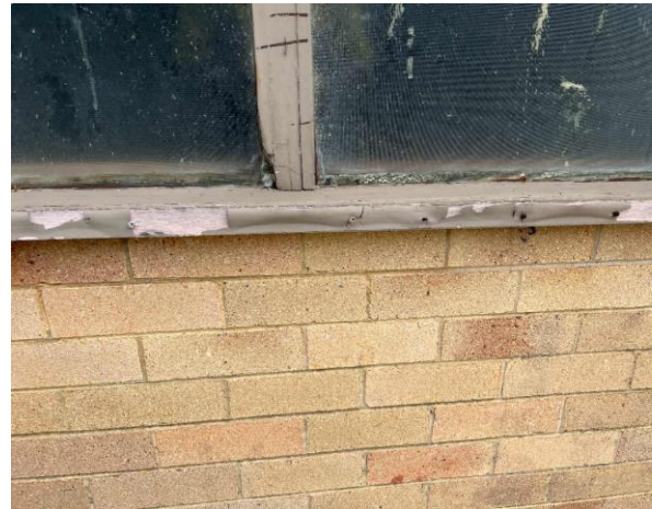
Line ID 43.1: External, Project Coordinators Residence, Rear Garage, Timber Window Frames, Light Brown Paint - Lead Detected (0.22% w/w)
