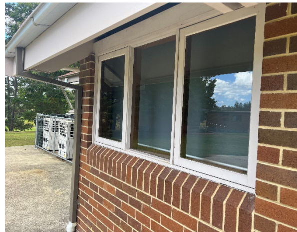
Line ID 43: Internal, Pool House, Throughout, Window Frames, Window Caulking - No Asbestos Detected
