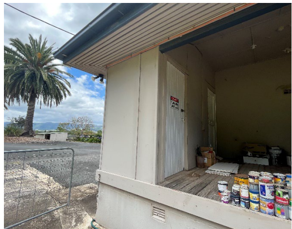
Line ID 54: External, Workshop and Silo, Maintenance Shed and Offices, Wall Linings, White Paint - Lead Detected (3.2% w/w)
