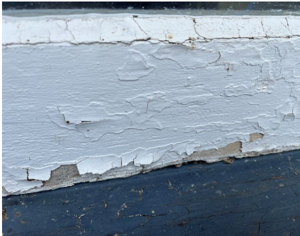
Line ID 16.1: External, Workshop and Silo, Maintenance Shed and Offices, Timber Windows Throughout, Window Caulking - No Asbestos Detected
