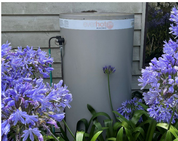
Line ID 61: External, North Residence, Verandas, Hot Water Unit, Insulation Material - Suspected SMF
