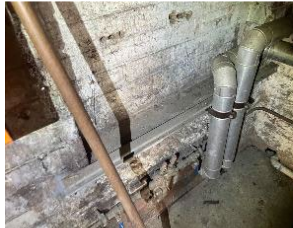
Line ID 56: Internal, Accommodation Building, Boiler House, Walls, White Paint - Lead Detected (0.02% w/w)
